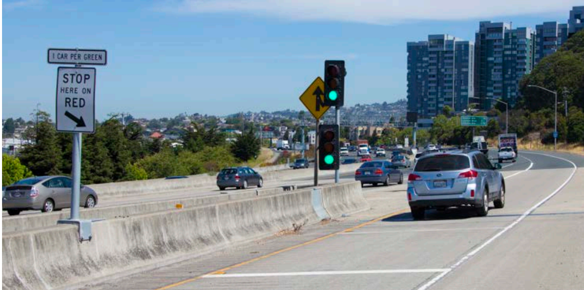
Figure 2 Typical single lane metered on-ramp on I-80 SMART Corridor (Caltrans Press Conference, 2016)
