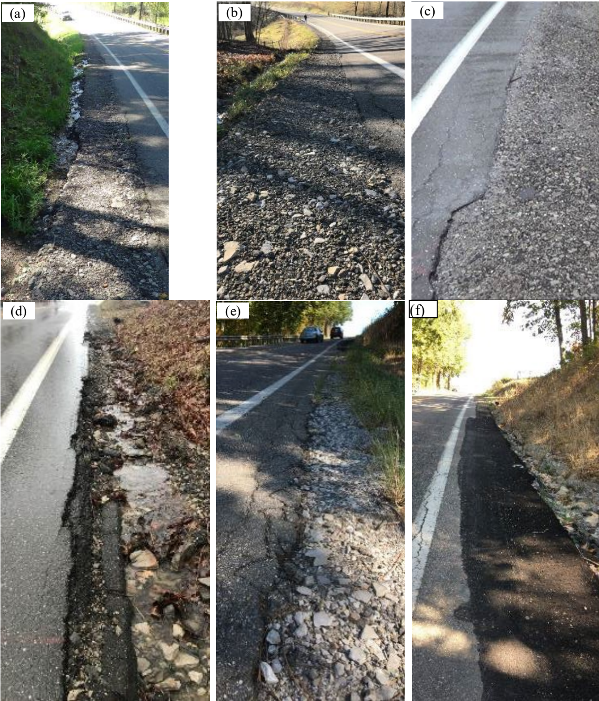
Figure B.9 Pictures from section two evaluation after: a. One month b. Four months c. Six months (first part of section) d. Six months (second part of section) e. One year f. 3 months (Repaired part
