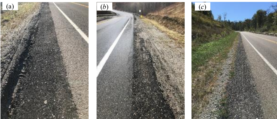
Figure B.16 Pictures from section eight evaluations: a. One month b. Four months c. One year
