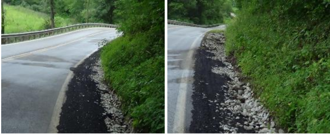
Figure A.5 Picture of repairs on SR 148
