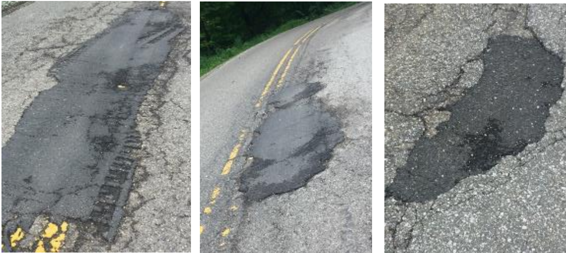
Figure A.5 Picture of repairs on SR 255
