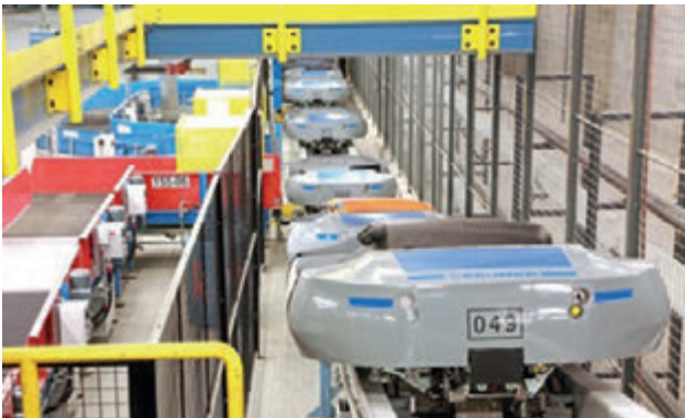
FIGURE 5.3 Automated baggage sorting and screening systems
