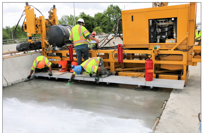
Installation of a UHPC overlay. Source: FHWA
