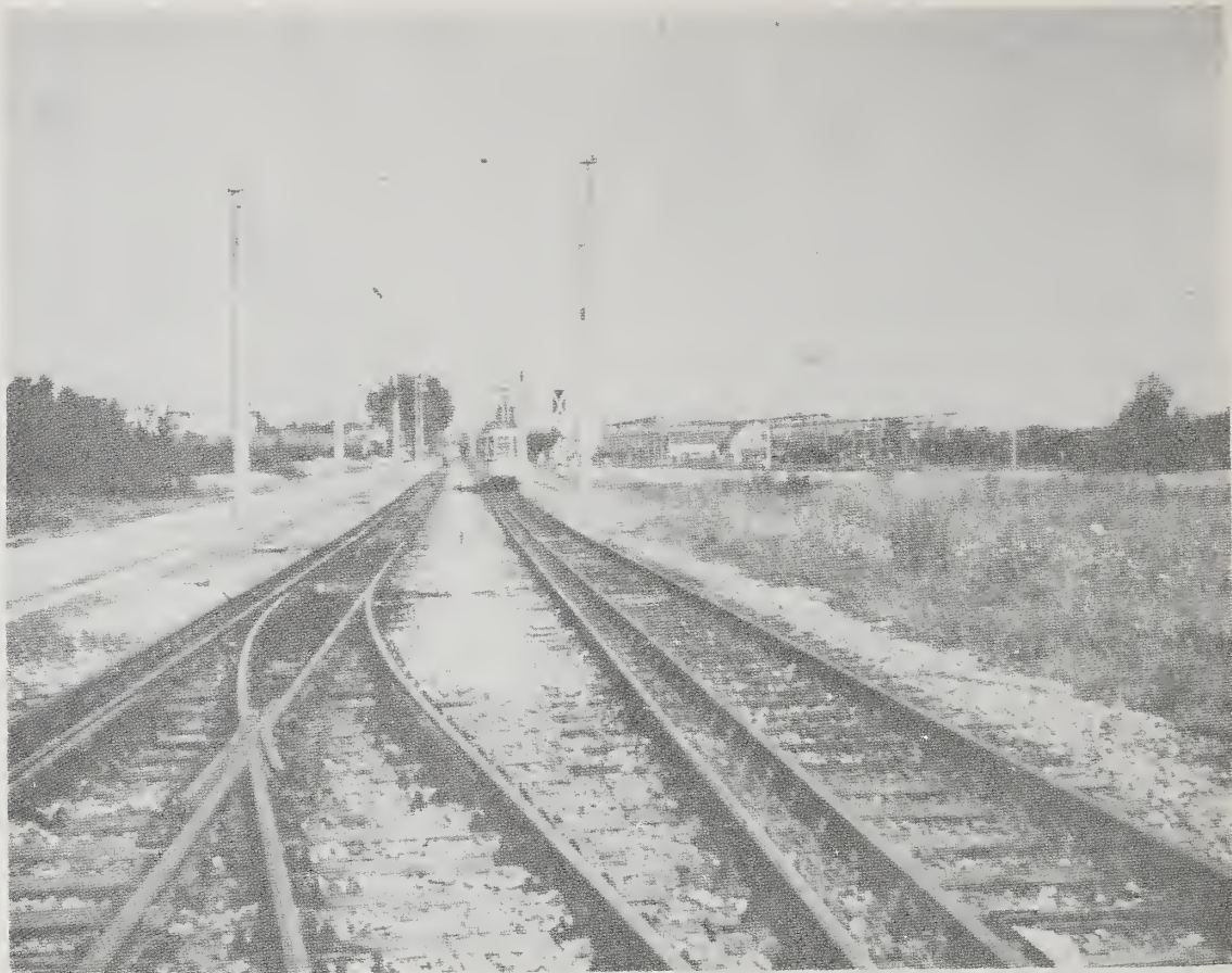
Figure 18. Joint Use Track, Mixed Gauge, in Stuttgart
