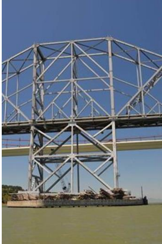
Figure 51. Photo. Pier 3 of the 1958 Carquinez Bridge (2003 bridge in background).
