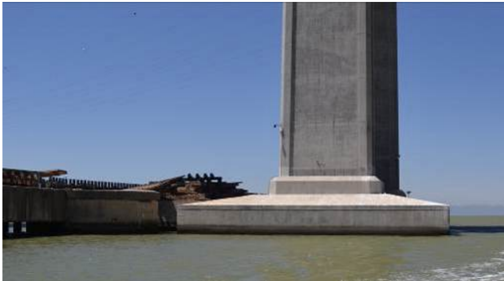
Figure 61. Photo. Tower 3 pile cap.
