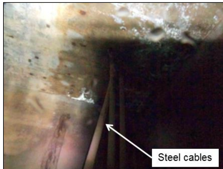
Figure 37. Photo. Above water view of steel cables.
