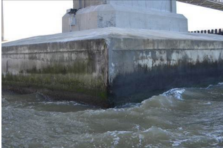
Figure 62. Photo. Tower 3 pile cap close-up.
