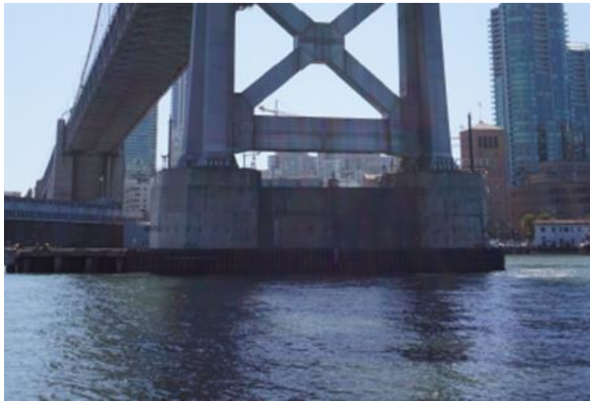
Figure 76. Photo. Pier W2 viewed from the east.
