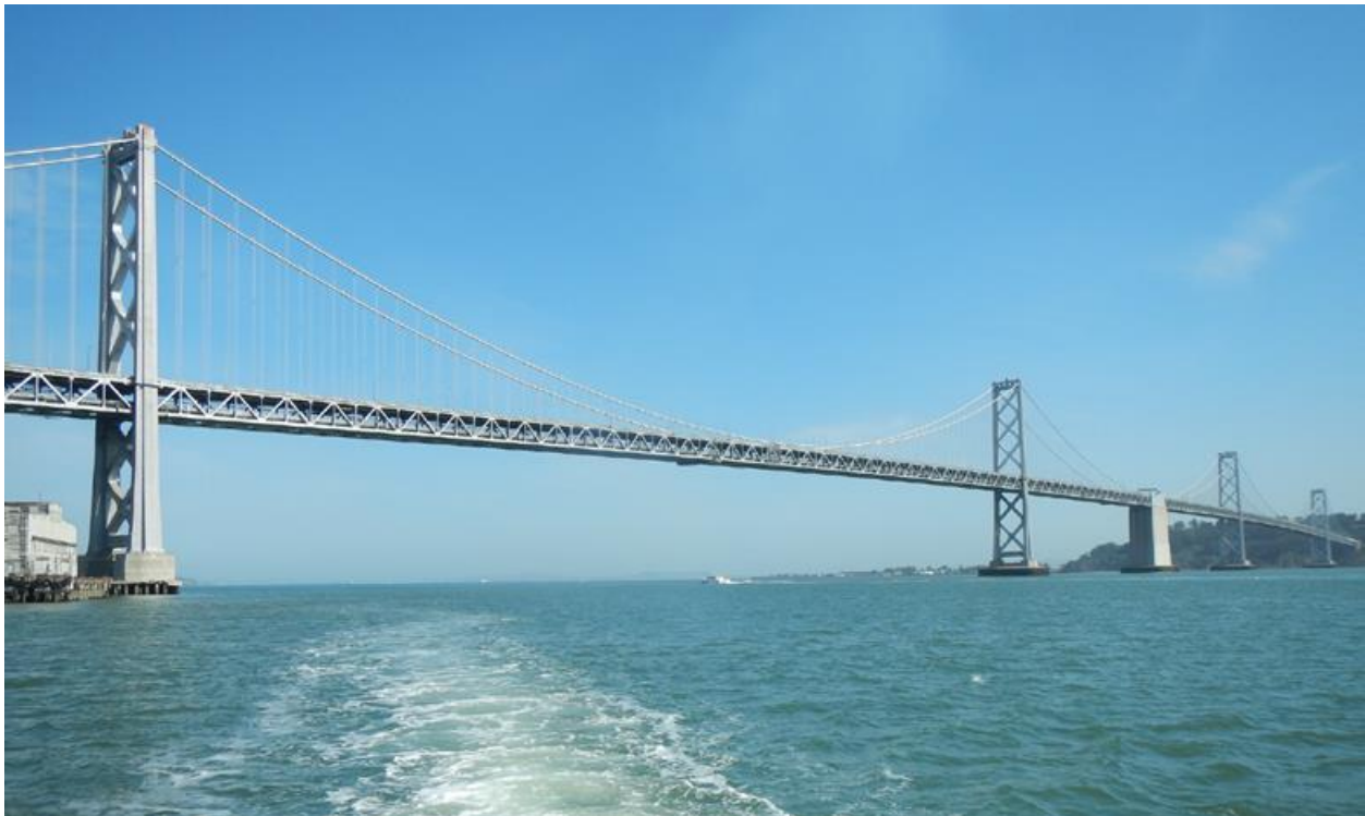
Figure 70. Photo. SF-OBB viewed from the south.
