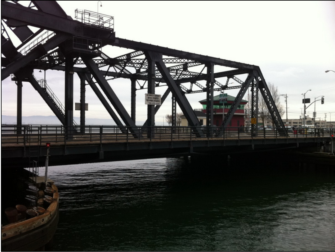
Figure 71. Photo. Third Street Bridge.
