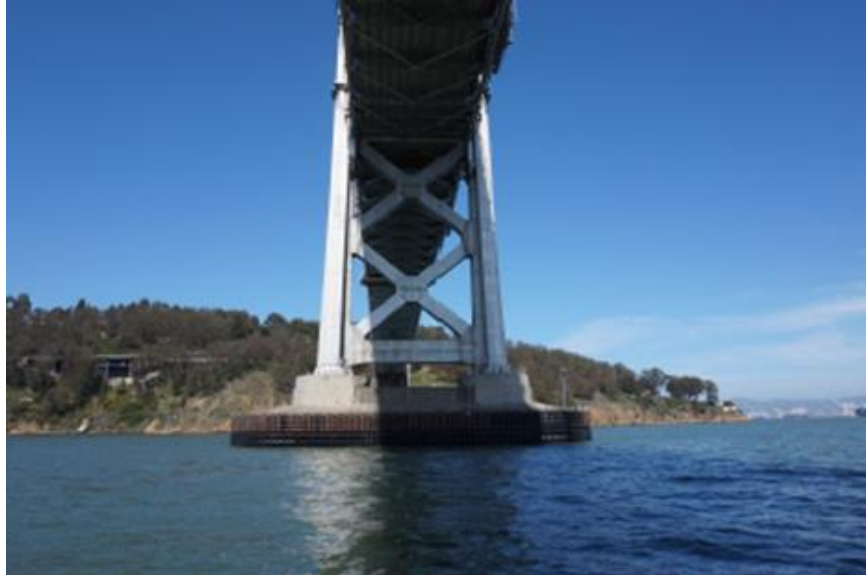
Figure 77. Photo. Pier W6 viewed from the west.
