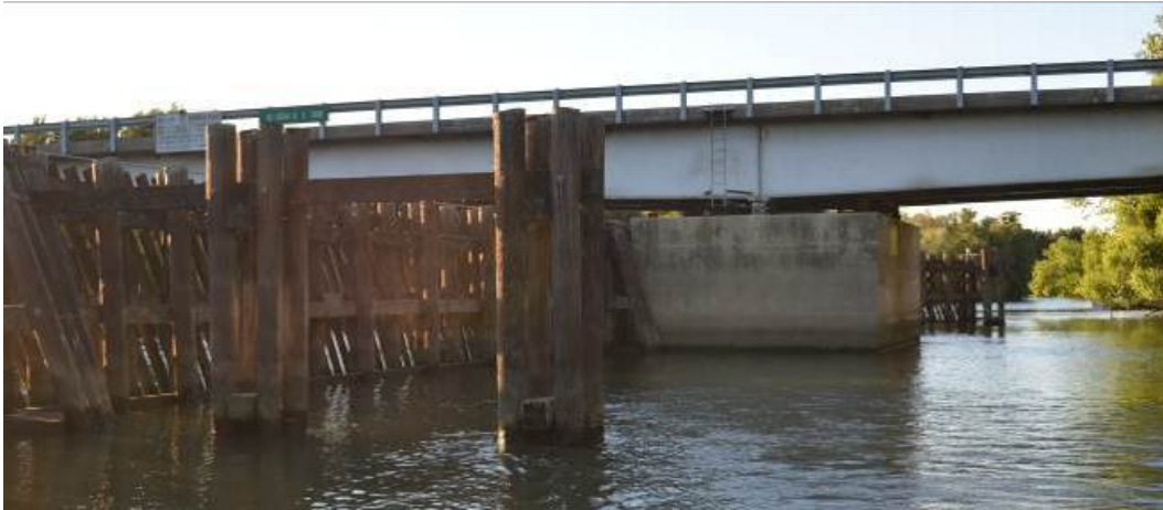
A. Looking north behind the timber fender.
