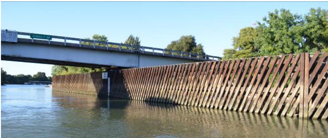
B. Looking north from the main channel.
