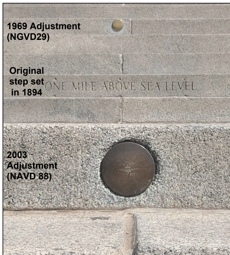
Figure 4.5. Colorado State Capital steps showing multiple adjustments made to the one mile above sea level location.
