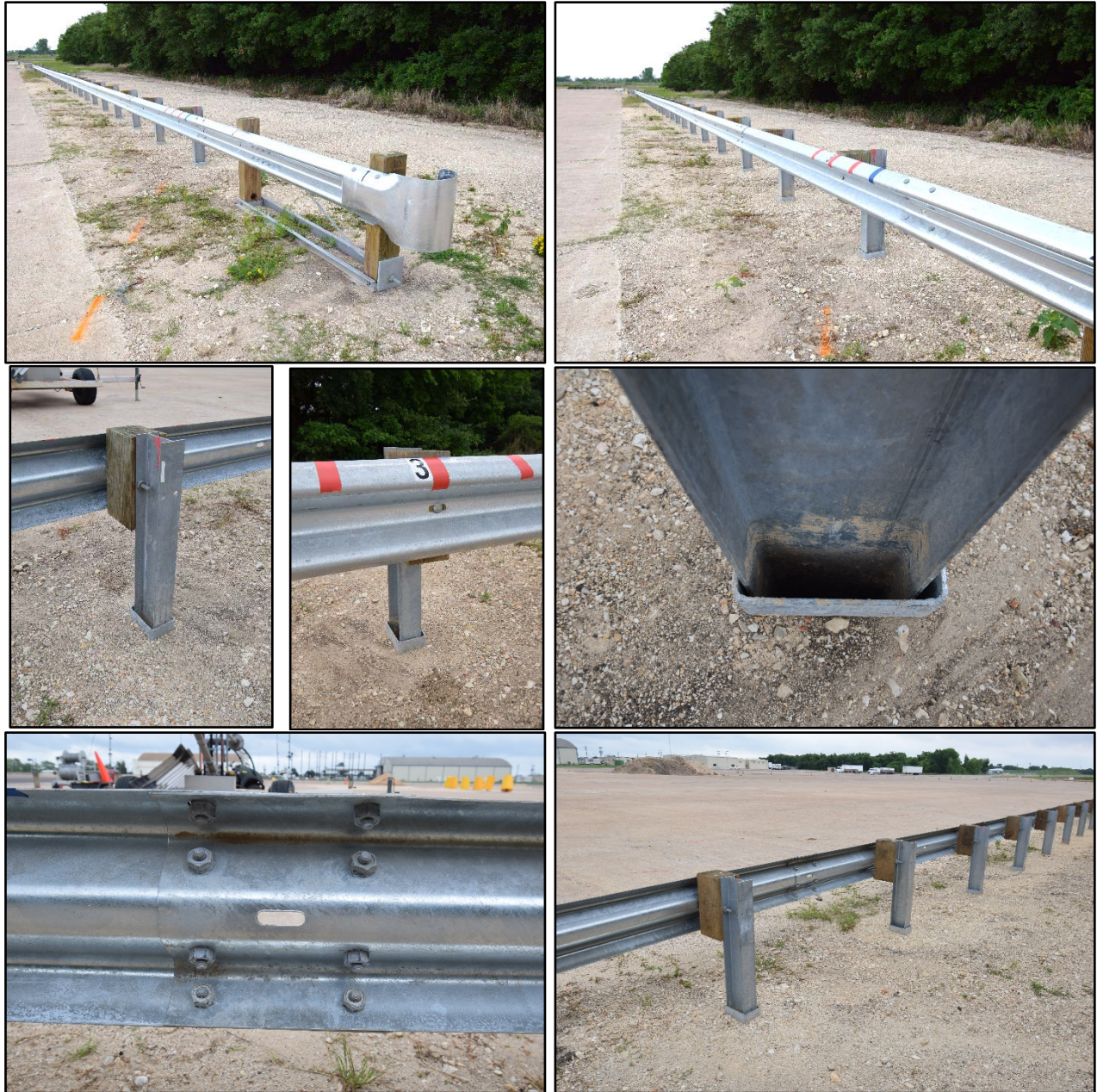
Figure 4.2. 31-inch Guardrail Terminal with Steel Posts in Steel Sleeves prior to Testing.
