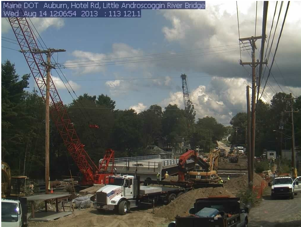
Figure 27. Photo. Webcam view of sliding operation on August 14, 2013.
