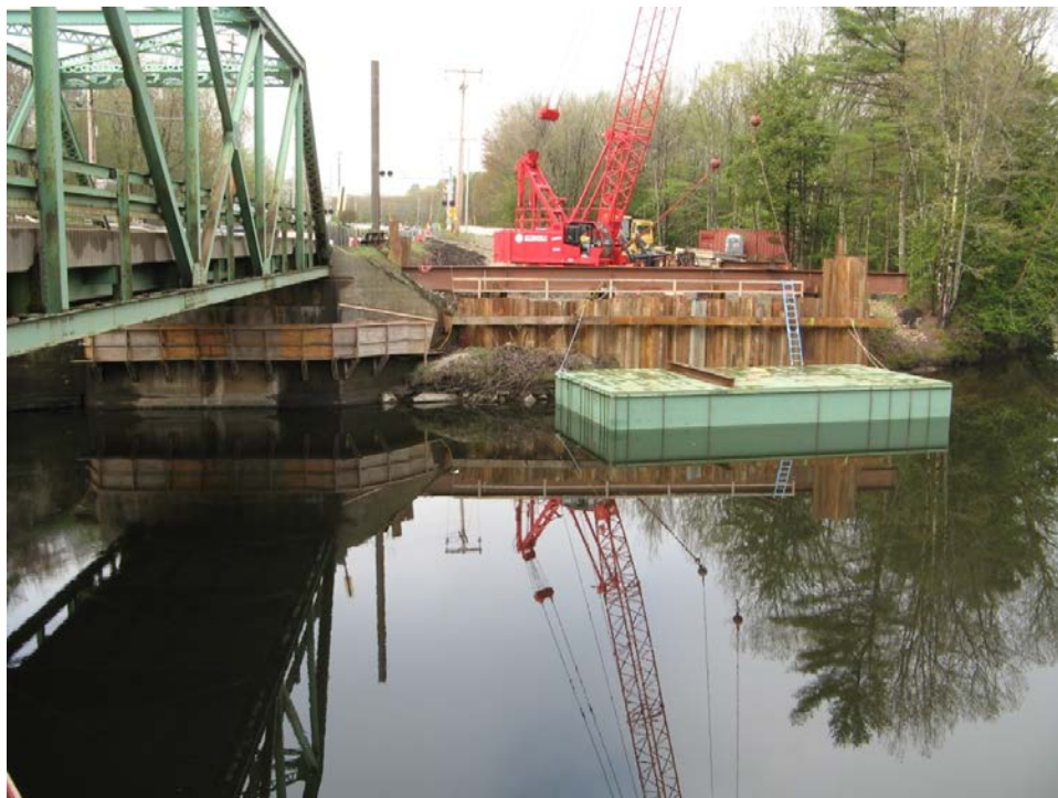
Figure 11. Photo. Sheetpiling working platforms for existing substructure in place.
