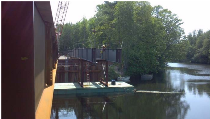
Figure 13. Photo. Girder launching and installation
