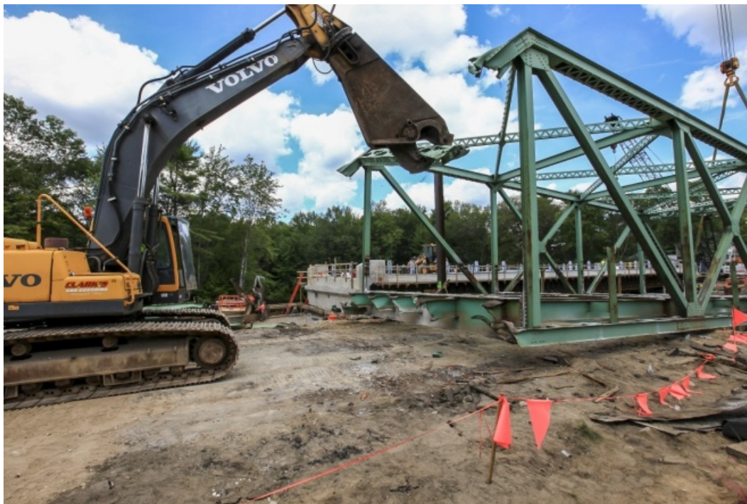
Figure 19. Photo. Old structure being demolished at site.
