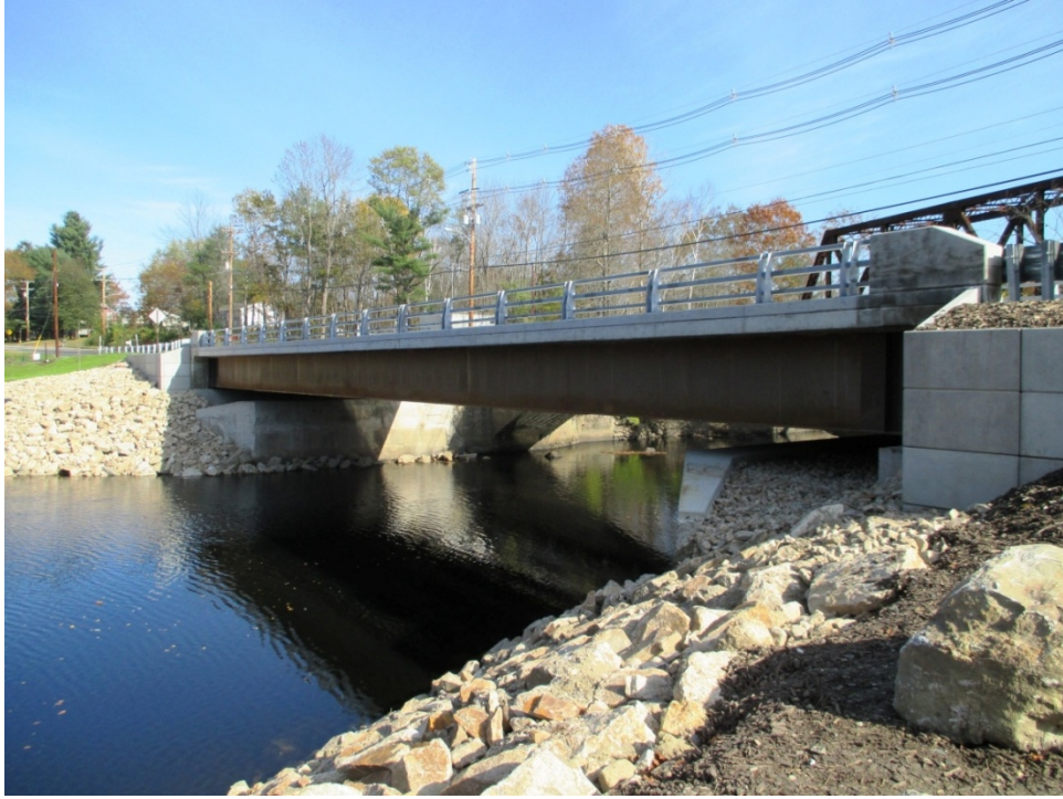
Figure 34. Photo. Elevation view of completed bridge.
