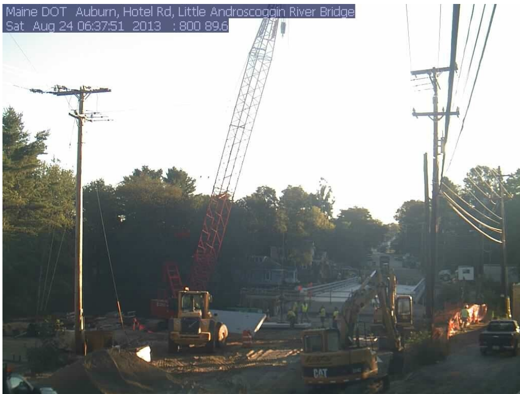
Figure 28. Photo. Installation of precast approach slabs.
