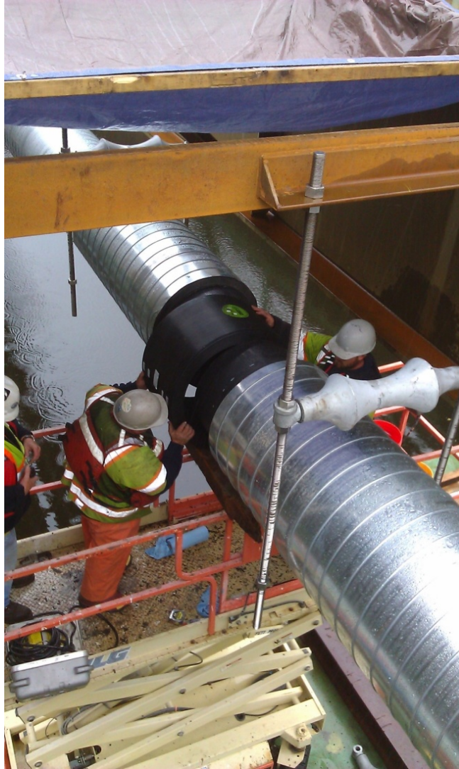
Figure 29. Photo. Utility installation.
