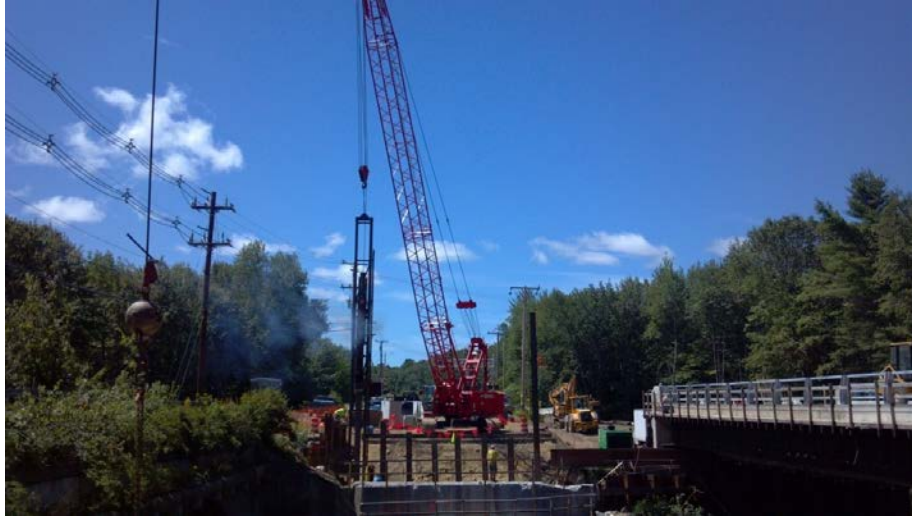
Figure 12. Photo. Pile driving for temporary support structure.
