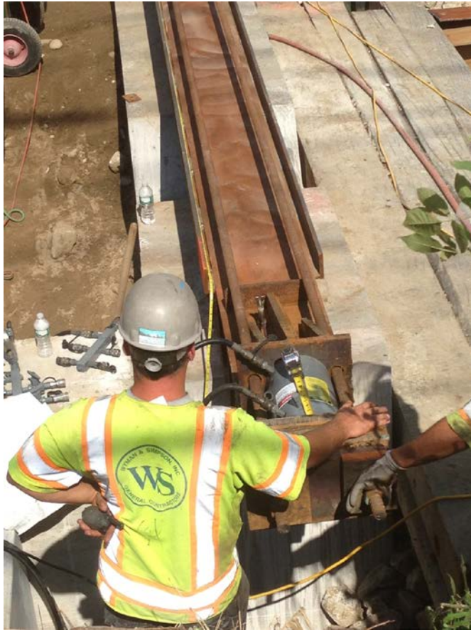
Figure 25. Photo. View of end anchorage.
