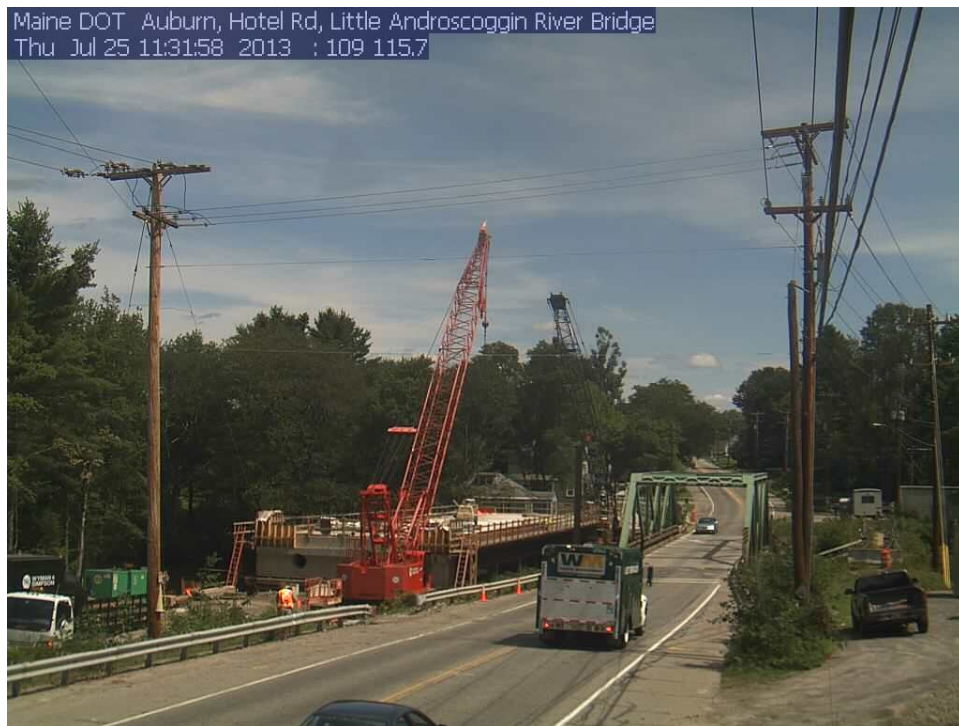
Figure 16. Photo. View of new superstructure in relation to old structure.
