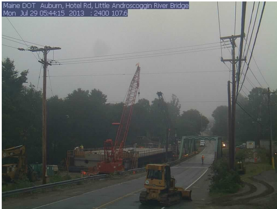
Figure 18. Photo. Roadway closure in process.
