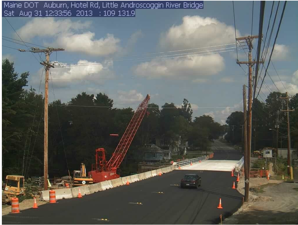
Figure 32. Photo. Road opened for traffic use.
