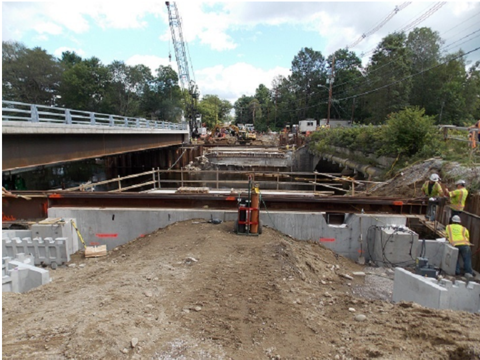
Figure 23. Photo. View of both abutments and anchor beam in foreground.
