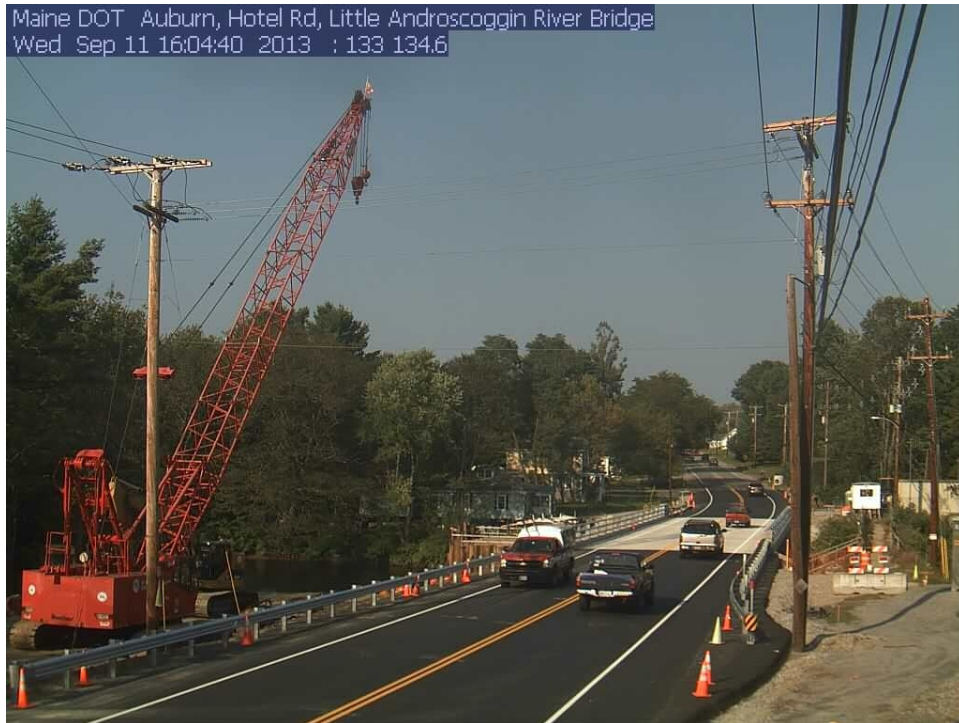
Figure 33. Photo. Guiderail installed, pavement striped, and new bridge in place.
