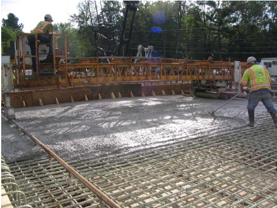
Figure 15. Photo. Concrete placement.
