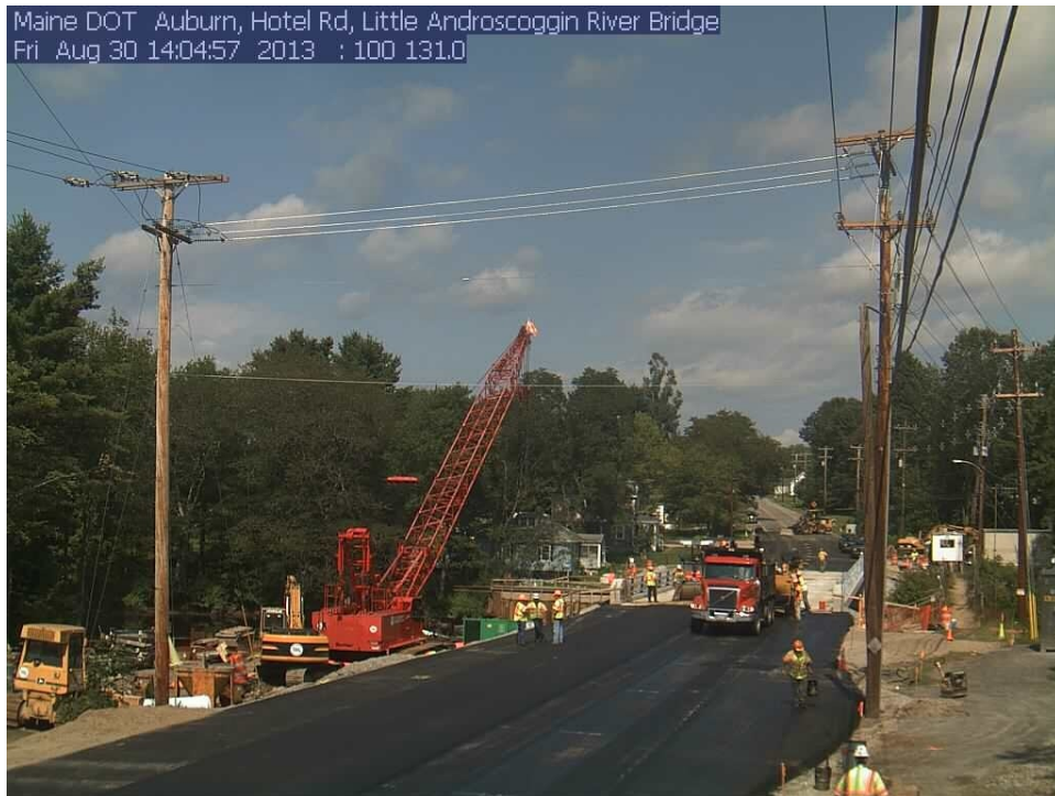
Figure 31. Photo. Placement of asphalt material for surface courses.
