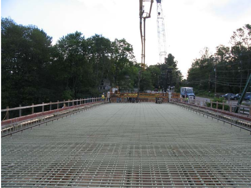
Figure 14. Photo. View of GFRP rebar prior to placement off concrete.
