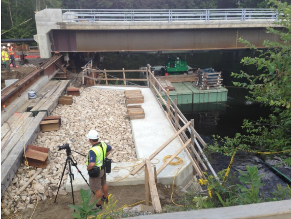
Figure 24. Photo. View of slide operation from the existing abutment side.
