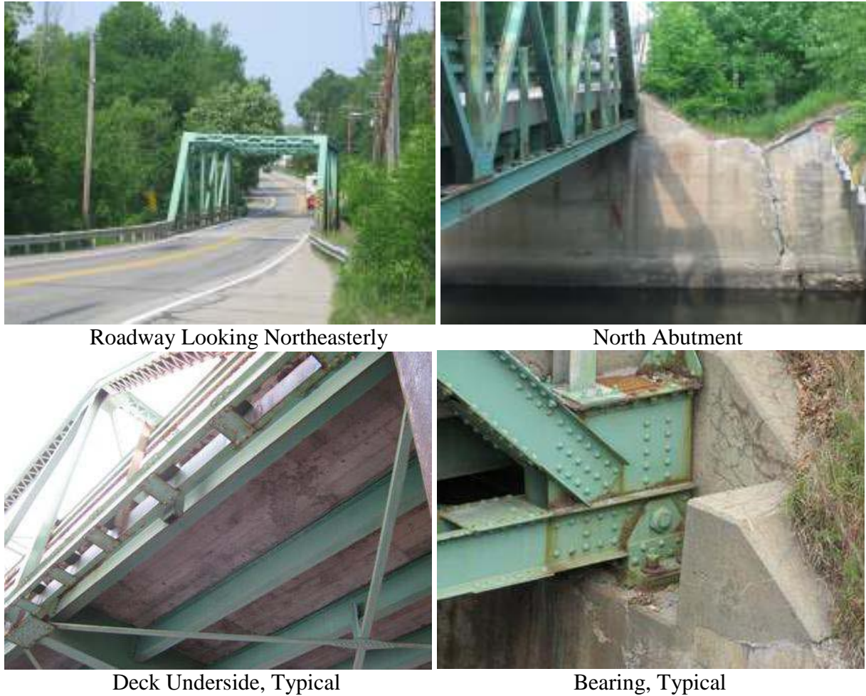
Figure 3. Photos. Photographs of old structure.
