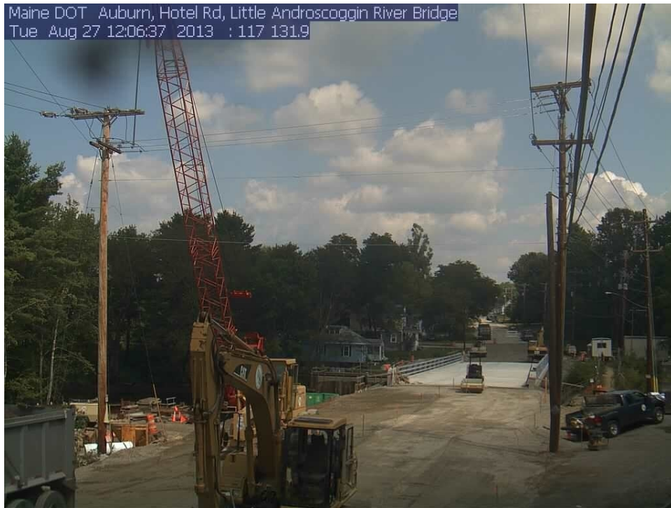
Figure 30. Photo. Preparation of subgrade for approach roadways.
