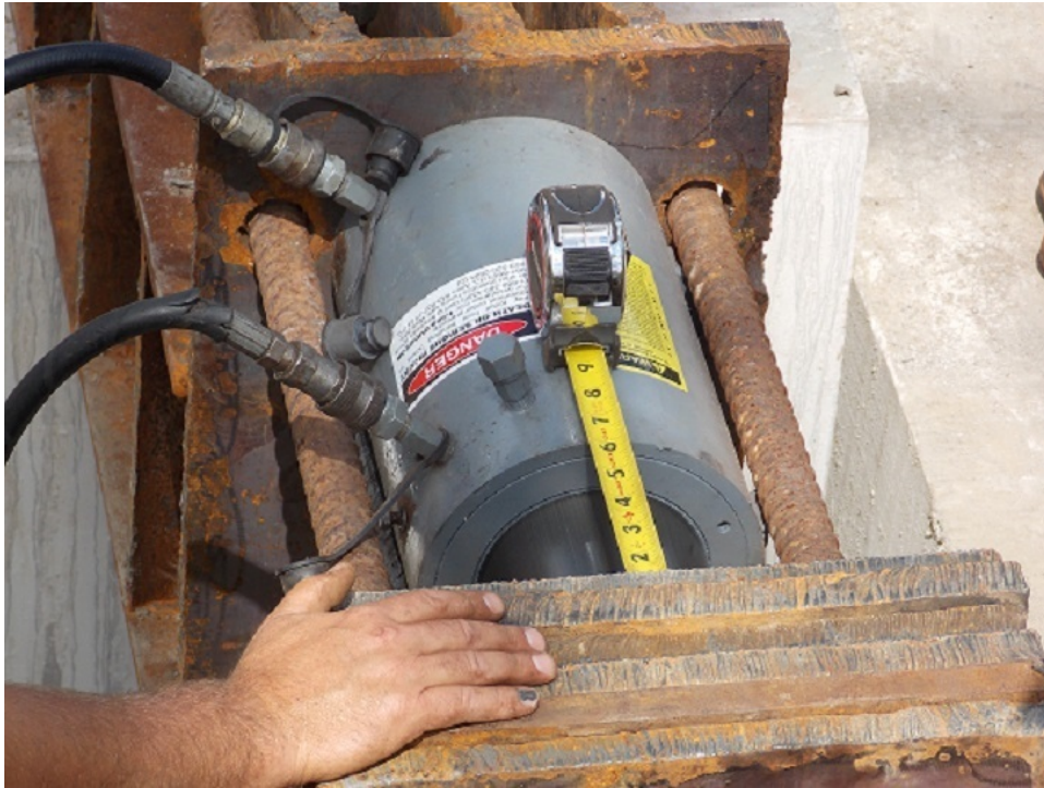
Figure 26. Photo. Close-up of Dywidag rods, jack, and jacking plates.
