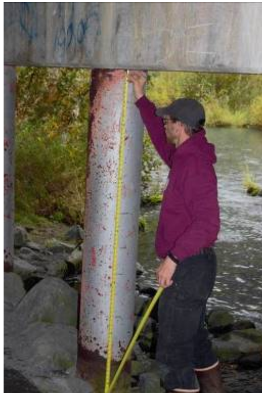
Figure 2: (a) Schematic of typical pile with sensor spacing details (b) Pile preparation
