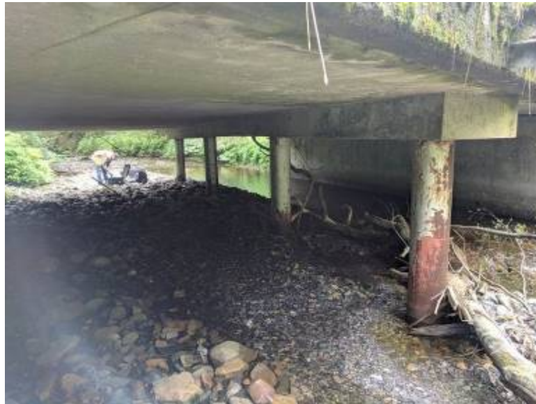
Figure 24: Lake creek pile
