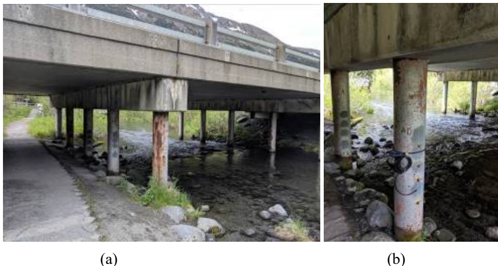
Figure 18: (a) Portage creek (b) Instrumented pile
