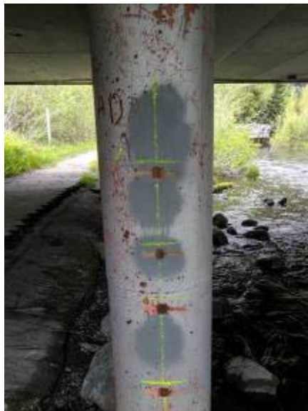
Figure 3: Surface Preparation
