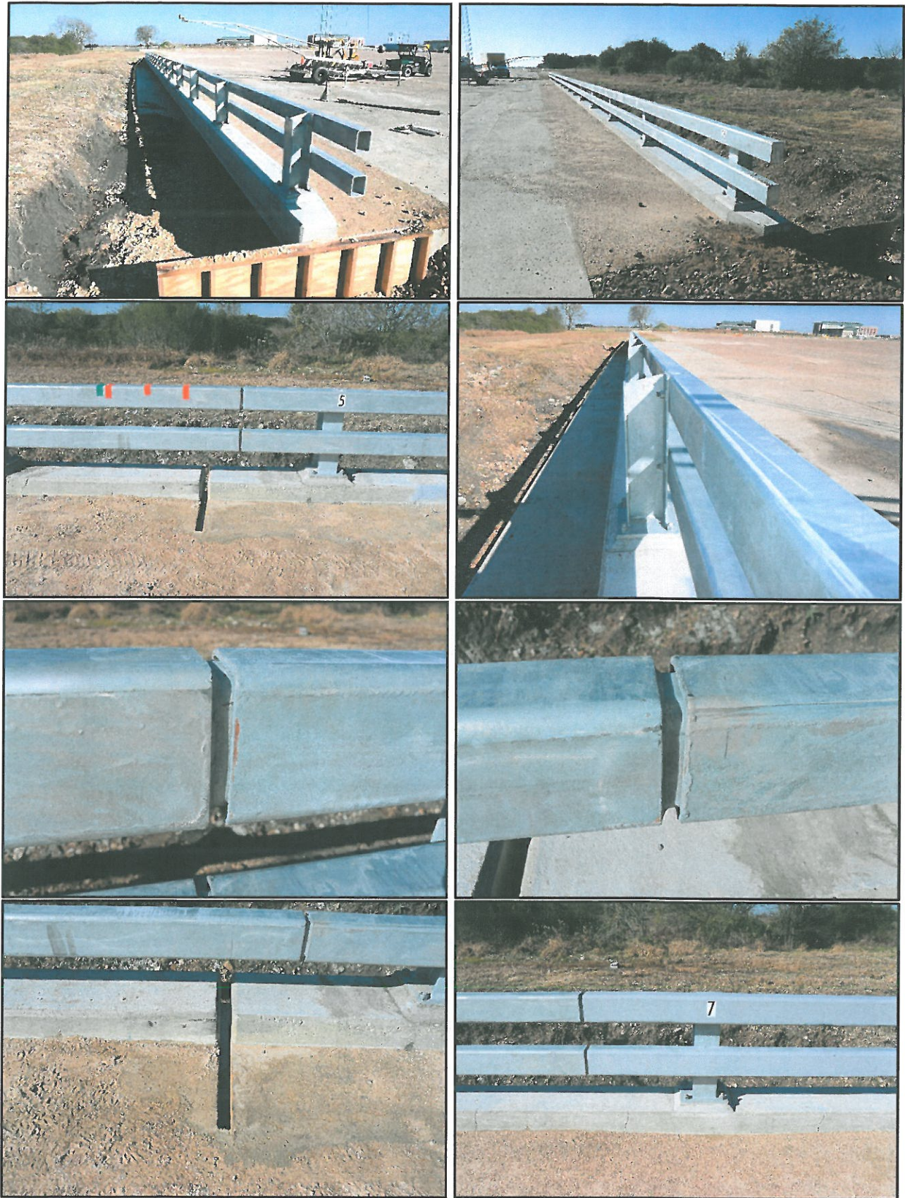
Figure 2.2. 2019 MASH 2-Tube Bridge Rail prior to Testing.
