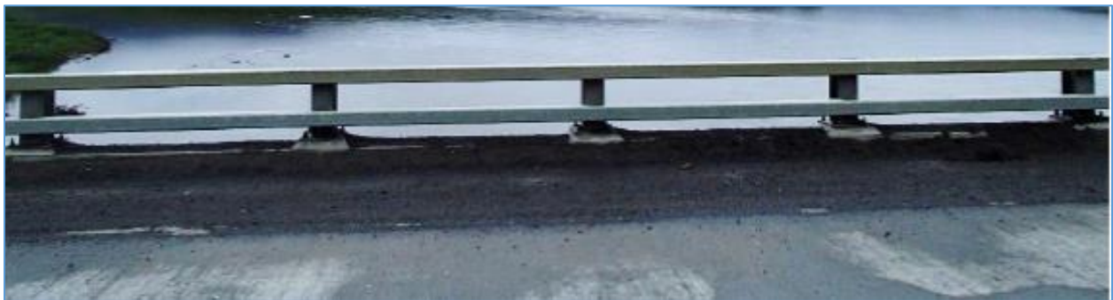
Figure 2.2 Atigun River No. 2 Bridge (Alaska DOT&PF Bridge Section, 2018)
