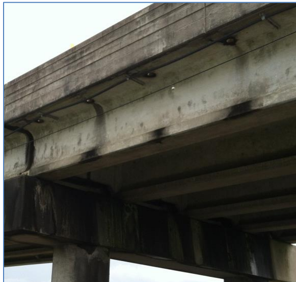
Figure 9: Outside edge of bridge showing concave configuration which traps an air pocket when a wave strikes it and potentially increases lateral loads. 19
