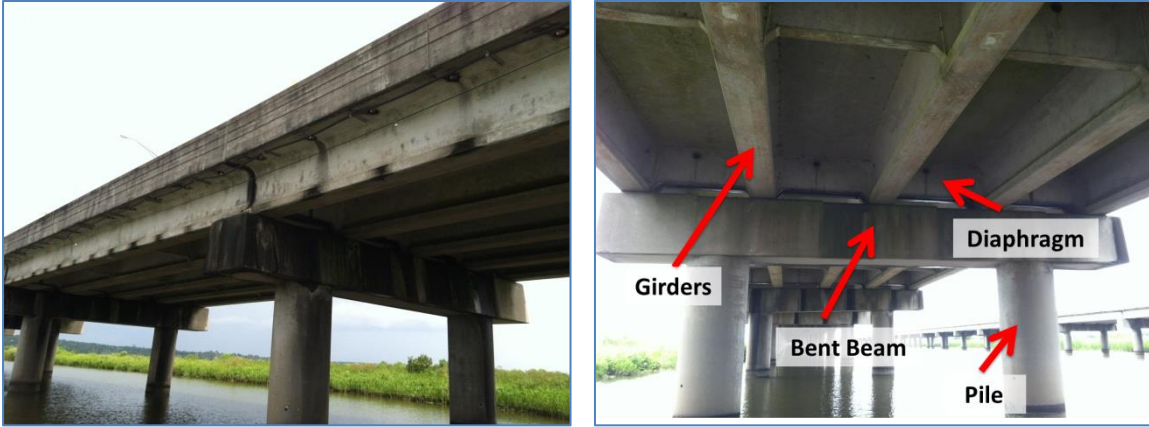
Figure 3: Photographs of a typical bridge section of the I-10 Bayway Bridge from below. 8
