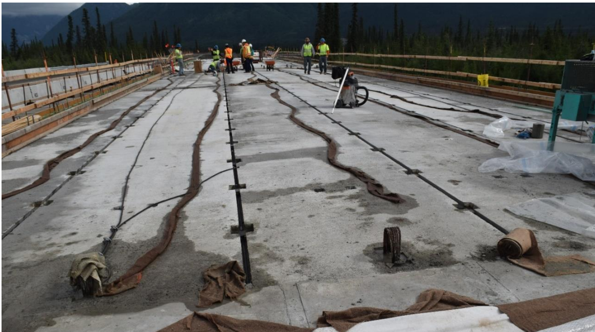
Figure G-9. Longitudinal keyways of bridge
