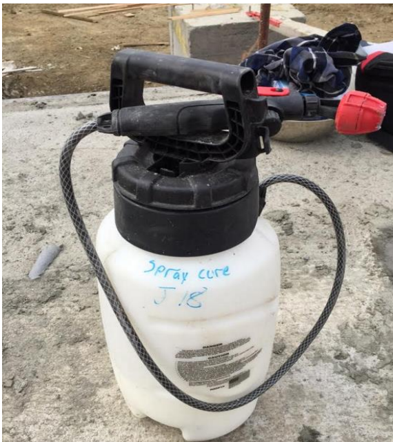
(a) Spray cure container
