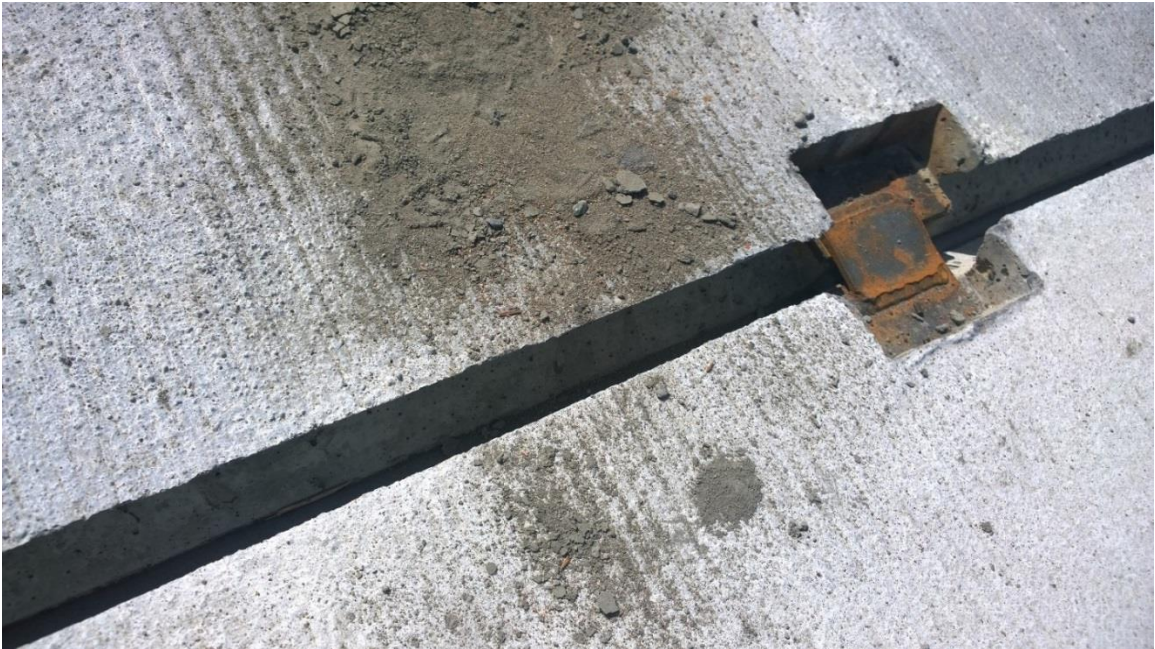
Figure G-12. Empty keyway just before grouting
