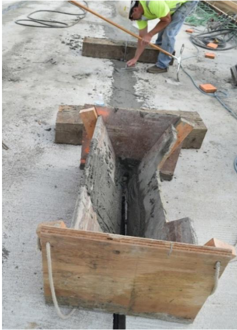
(a) Grout pouring form
