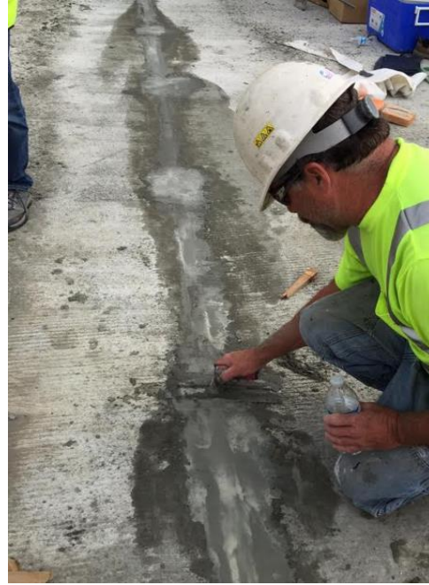
(b) Surface finishing with a trowel
