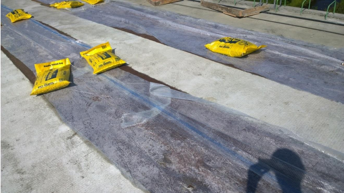
Figure G-15. Grout curing with wet burlap and plastic cover
