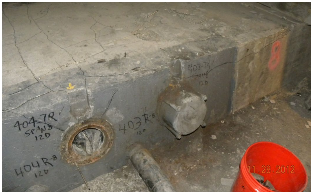
Figure 2-4 Cracked Concrete Anchor Block During De-tensioning
