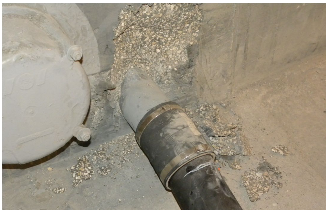
Figure 2-5 Rigid Steel Pipe Pull-out Resulting in Spalled Concrete
