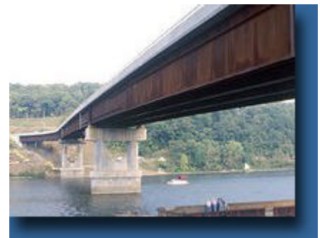
Photo 3.1.5 Ford City Bridge
