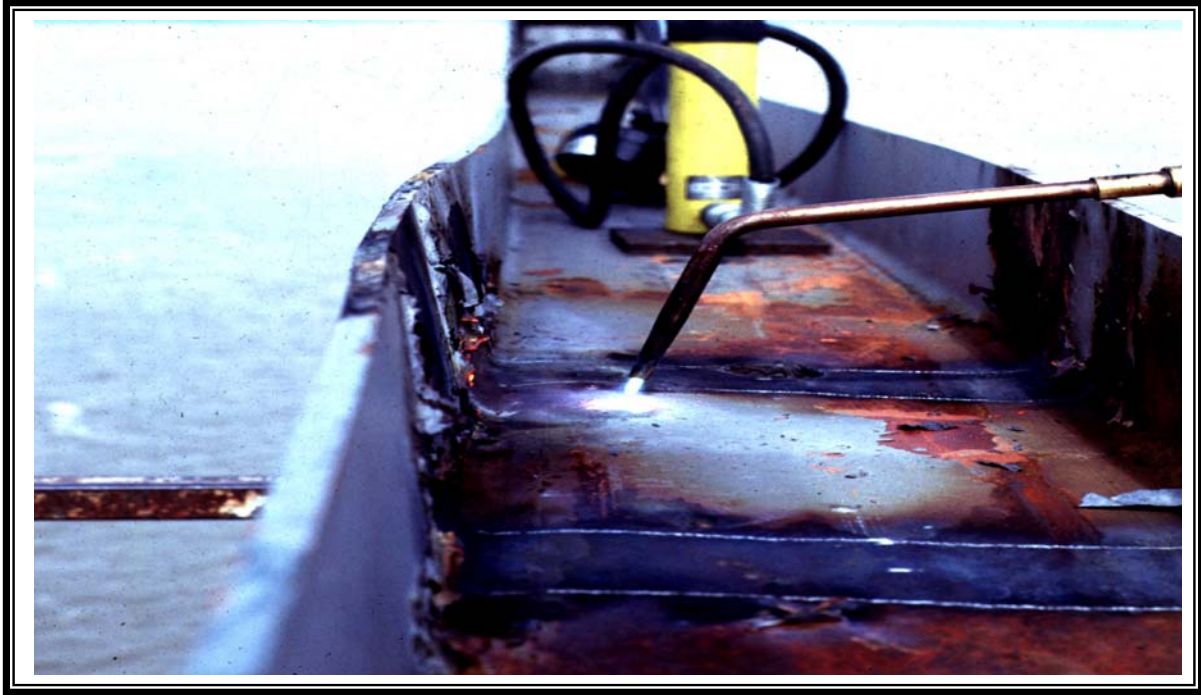
Figure 10. Strip heat in progress with a completed strip heat in the foreground.
