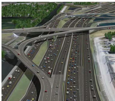
I-595 corridor roadway improvements.
