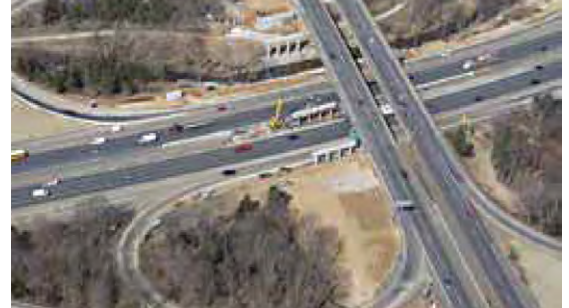
I-495 Capital Beltway high-occupancy toll lanes.
