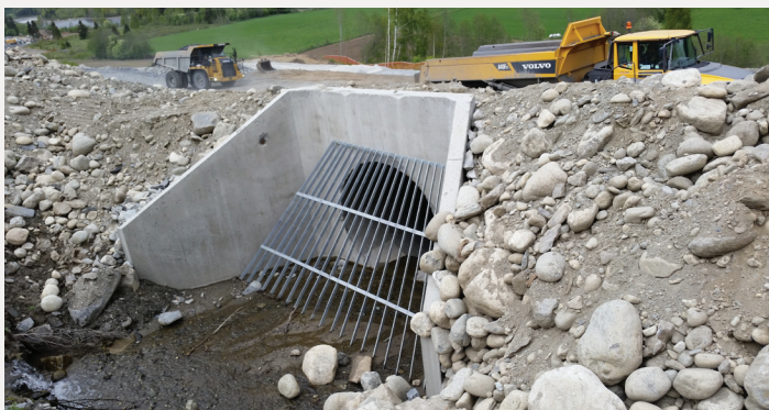
Figure 1 (Above): Debris screen at culvert in Norway. Photo credit: FHWA
