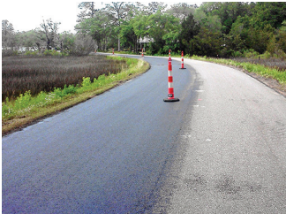
Charleston County, S.C. Figure 1. Asphalt rubber chip sealing
