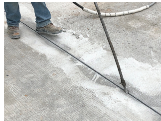
Dow Corning Figure 11. Joint sealing
