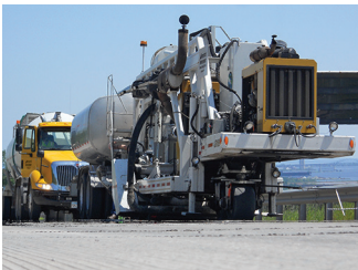
International Grooving and Grinding Association Figure 9. Diamond grinding
