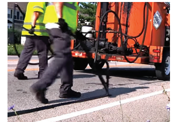
National Center for Pavement Preservation Figure 8. Crack sealing
