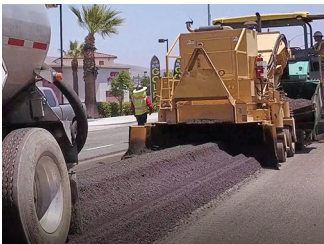
Pavement Recycling Systems Figure 5. Cold in-place recycling
