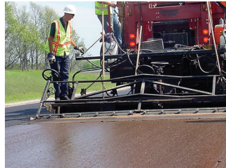
National Center for Pavement Preservation Figure 2. Micro surfacing
