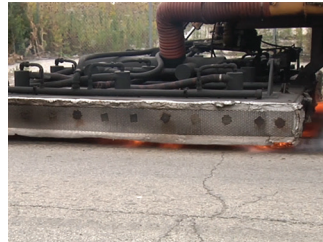
National Center for Pavement Preservation Figure 3. Hot in-place recycling
