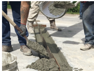
ACPA Figure 10. Partial-depth repair
