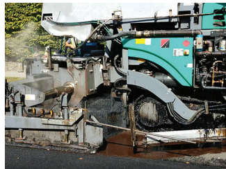
All States Materials Group Figure 6. Ultrathin bonded wearing course
