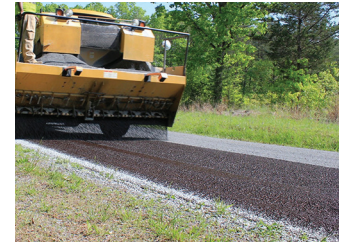
Slurry Pavers, Inc. Figure 4. Chip sealing
