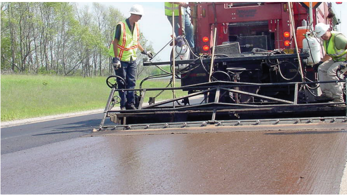
National Center for Pavement Preservation Figure 2. Micro surfacing
