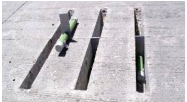
ACPA Figure 6. Dowel bar retrofit
