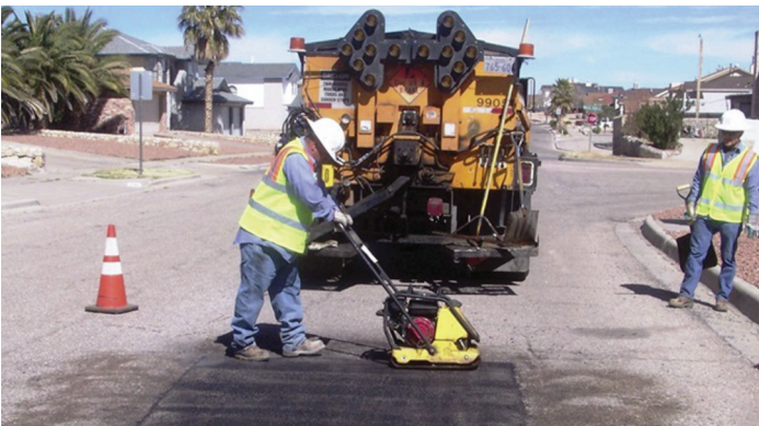
City of El Paso Figure 3. Asphalt patching
