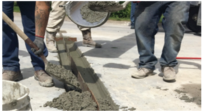
ACPA Figure 5. Partial-depth repair
