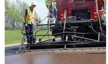
National Center for Pavement Preservation
