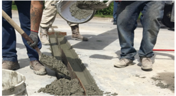
ACPA Figure 9. Partial-depth repair
