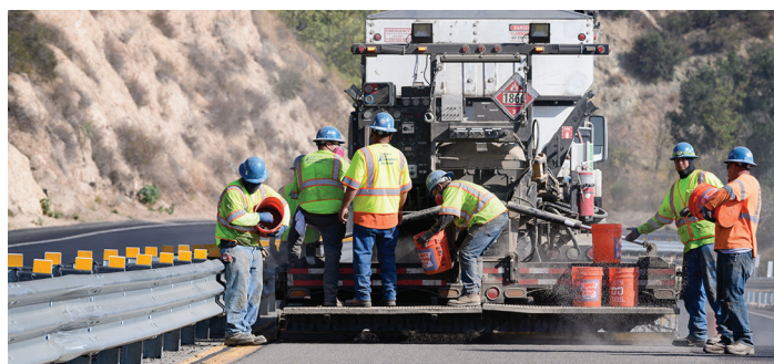
Kwik Bond Polymers Figure 3. High-friction surface treatment
