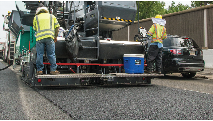
Tom Kuennen Figure 4. Open-graded friction course
