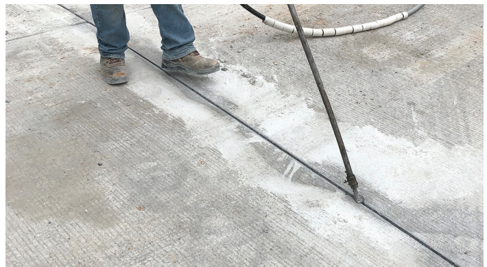
Dow Corning Figure 11. Joint sealing
