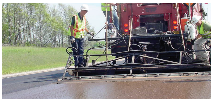
National Center for Pavement Preservation Figure 2. Micro surfacing
