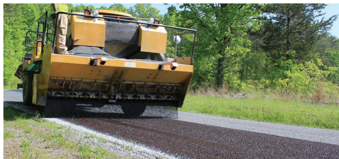
Slurry Pavers, Inc. Figure 1. Chip sealing
