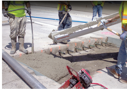
ACPA, used with permission Figure 12. Full-depth repair
