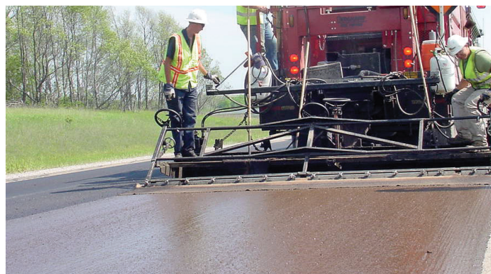
National Center for Pavement Preservation
