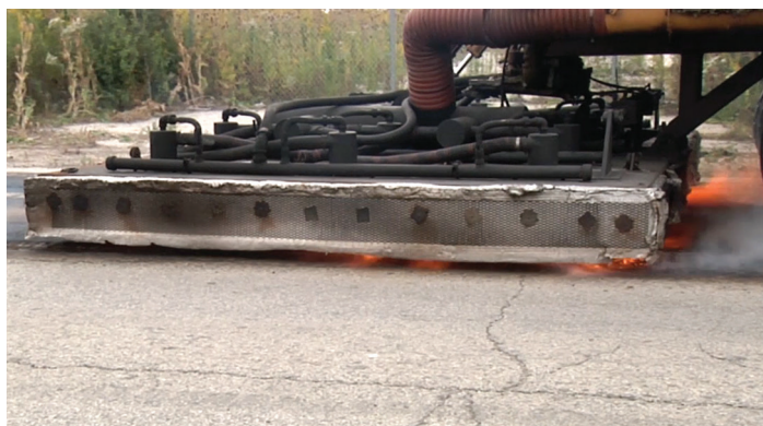
National Center for Pavement Preservation
