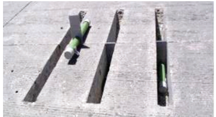
ACPA Figure 10. Dowel bar retrofit
