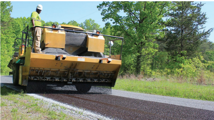
Slurry Pavers, Inc. Figure 6. Chip sealing
