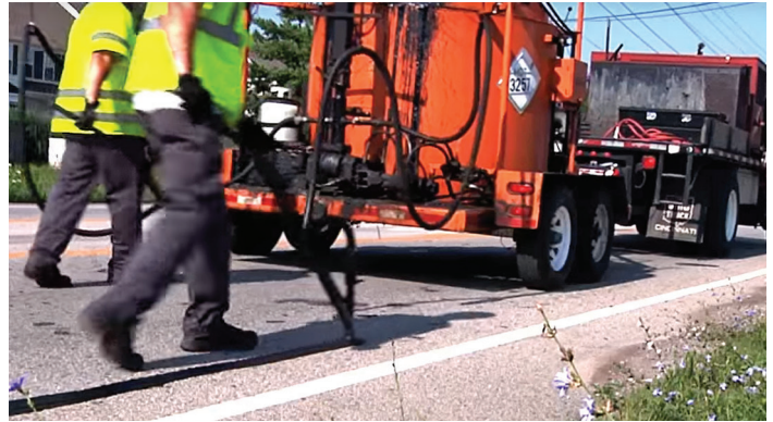
National Center for Pavement Preservation Figure 6. Crack sealing
