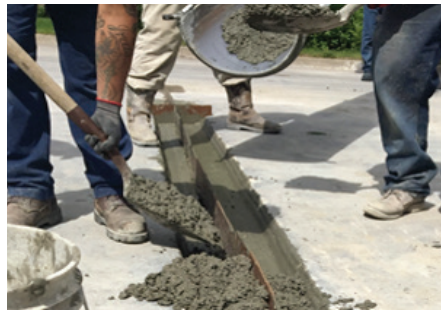
ACPA, used with permission Figure 9. Partial-depth repair
