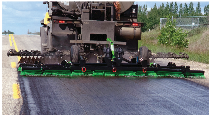
Saskatchewan Ministry of Highways and Infrastructure Figure 7. Scrub sealing
