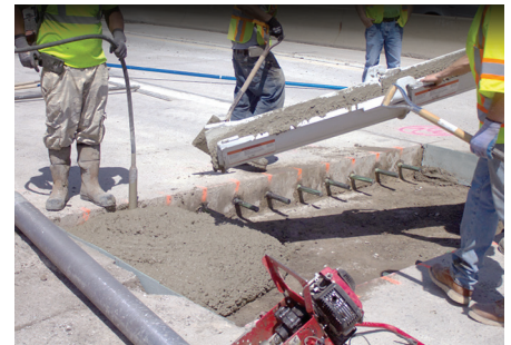
ACPA, used with permission Figure 10. Full-depth repair
