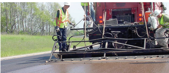
National Center for Pavement Preservation
