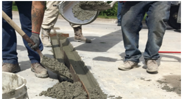
ACPA Figure 10. Partial-depth repair
