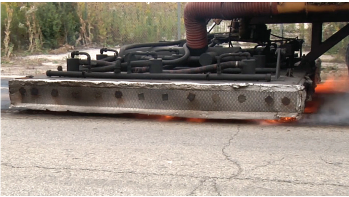
National Center for Pavement Preservation Figure 5. Hot in-place recycling
