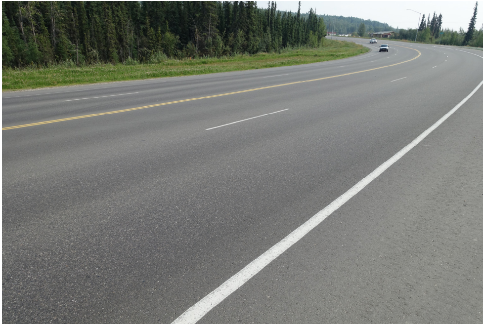
Figure 4.52 Richardson Hwy MP 337 Eielson AFB Intersection Improvements, PG 52-40, constructed in 2017
