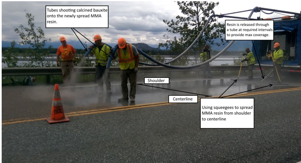
Photo 1: 2016 Application using Method 2 on Old Glenn Highway
