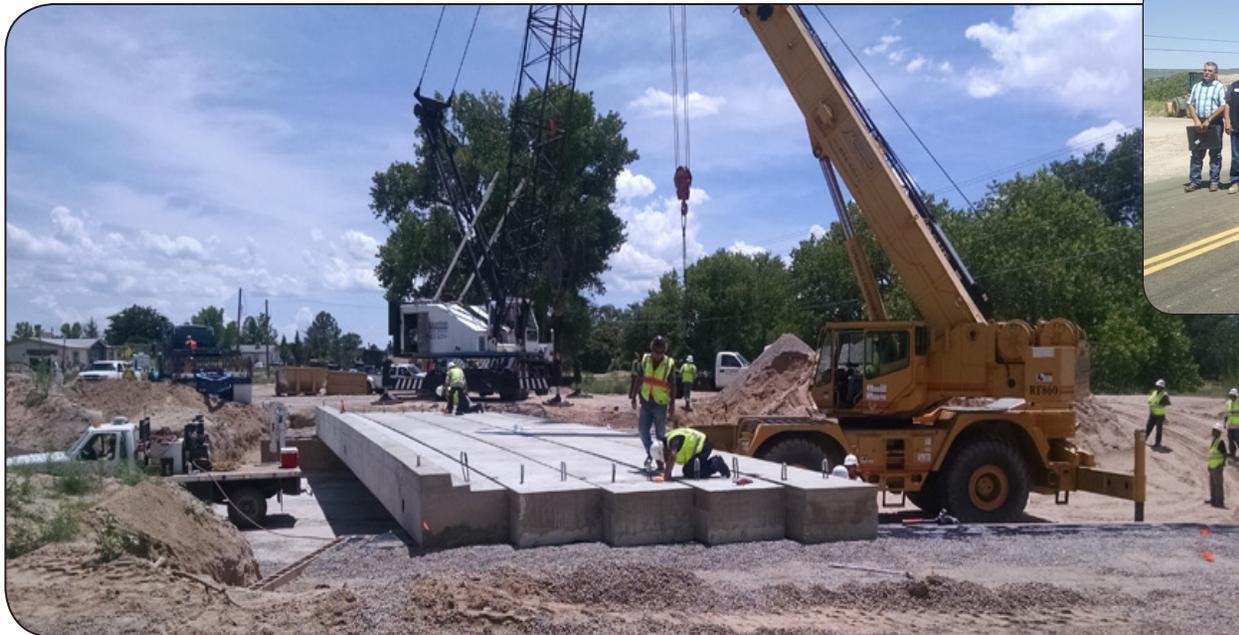
*Setting last girder into place and view of completed bridge*
