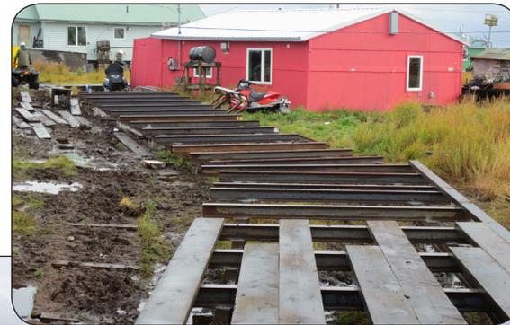
*Board installation on steel framing*
