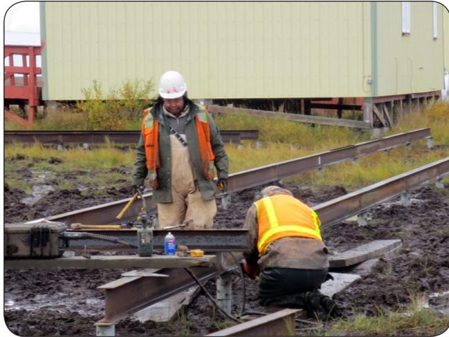
*Welding and assembly of boardroad framing*
