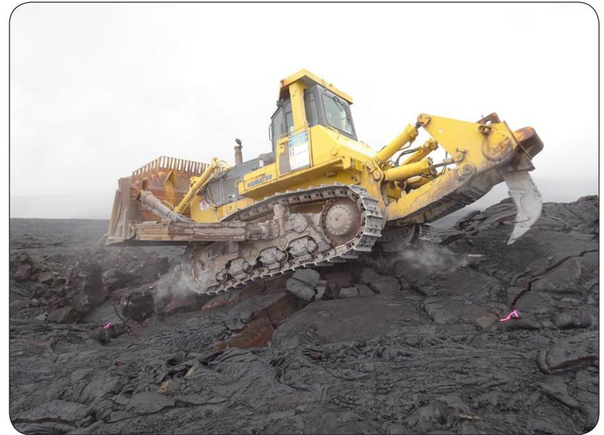
*Bulldozer as it begins to cut through the lava for the new roadway alignment*
