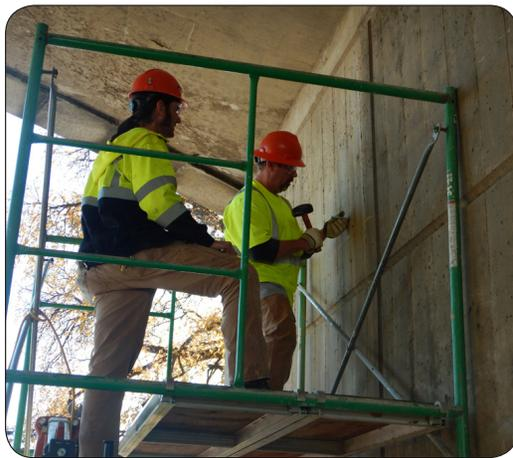
*Bridge Inspection staff drilling concrete test core samples from bridge abutment for in-depth investigation at Pentagon Reservation, Arlington, Virginia*
