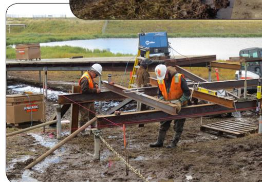
*Framing in preparation for welding*
