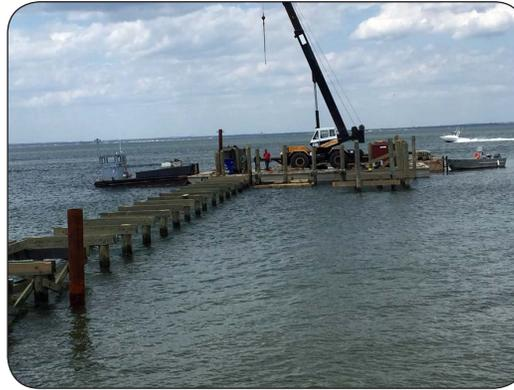
*Pile driving from construction barge*
