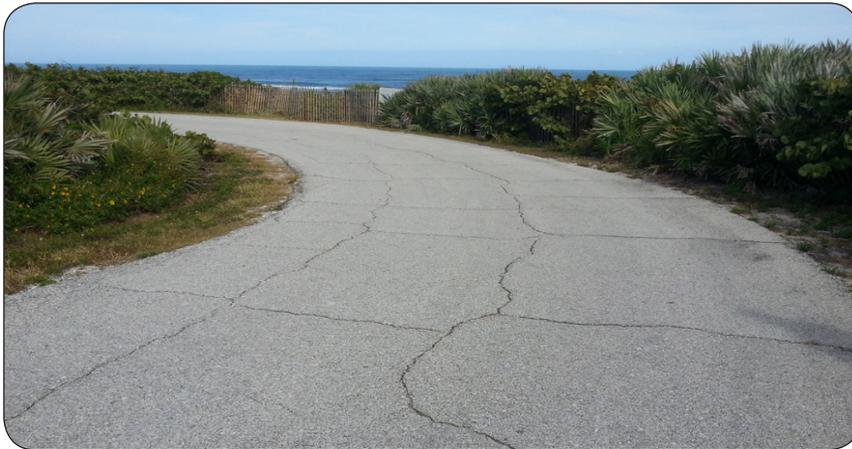
*View of a stretch of roadway condition showing visible cracks, a condition suitable for pavement preservation treatment as a low cost alternative to extend the life of the pavement at Canaveral National Seashore, Florida*
