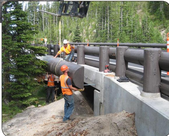
*Installing the first fascia logs to the bridge deck*
