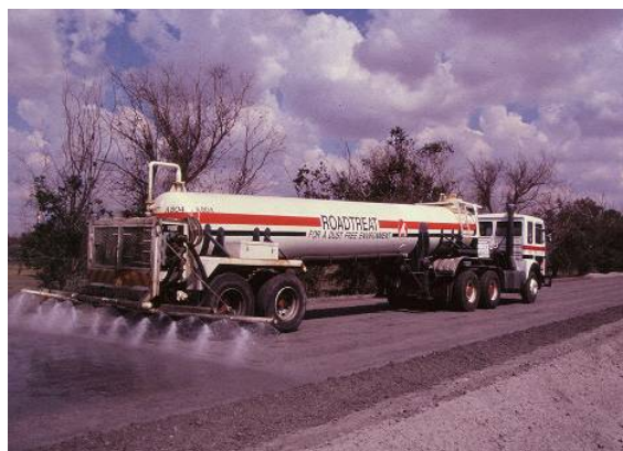
Figure 97. Photo. Road preparation to minimize environmental impact.
