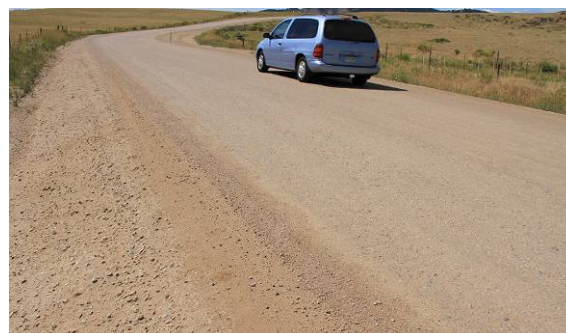
Figure 21. Photo. Road with good drainage.
