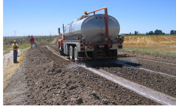
Figure 79. Photo. Spraying the additive.
