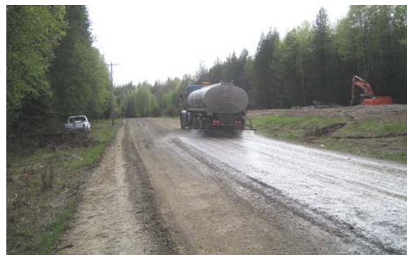
Figure 13. Photo. Spray-on treatment to well-prepared road.
