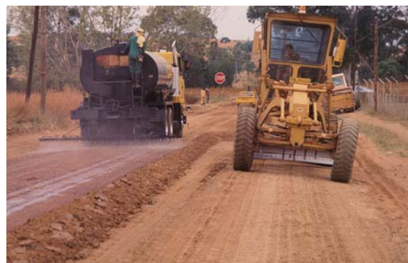
Figure 14. Photo. Mix-in treatment.
