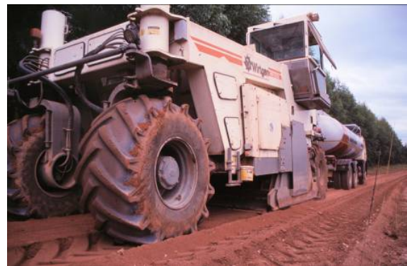
Figure 77. Photo. Full-depth recycler.
