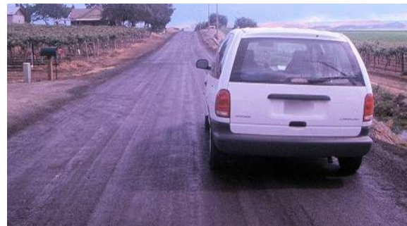
Figure 81. Photo. Completed road.
