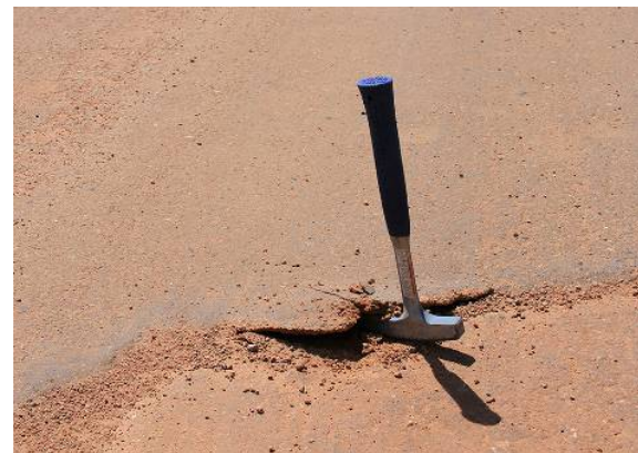
Figure 63. Photo. Effect of biscuit layer on treated surface.
