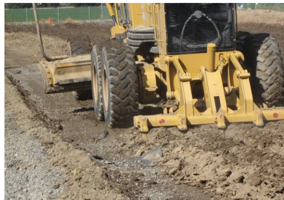
Figure 78. Photo. Ripping with a grader.
