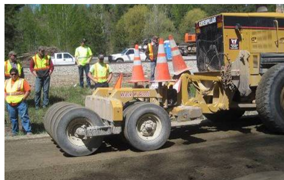
Figure 65. Photo. Grader-mounted roller.
