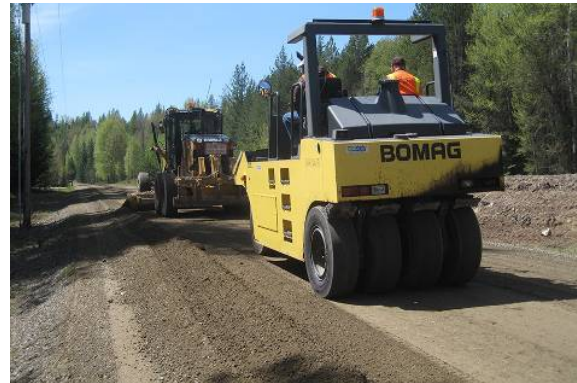
Figure 80. Photo. Compaction with rubber-tired roller.
