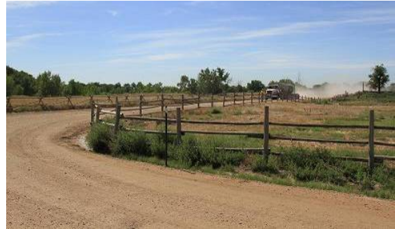
Figure 68. Photo. Very sharp curve.
