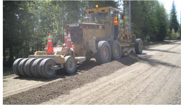
Figure 9. Photo. Grader maintenance.
