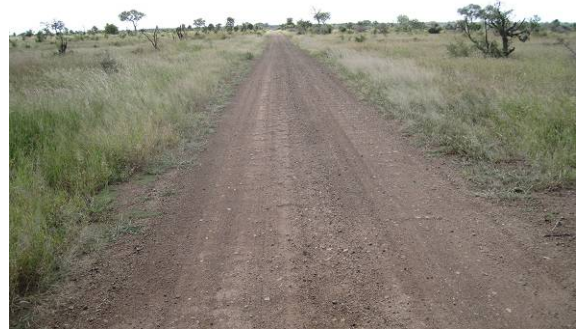
Figure 7. Photo. Low volume access road.
