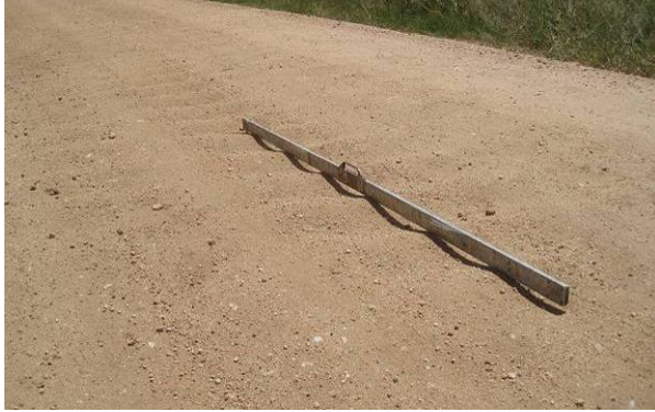
Figure 38. Photo. Washboarding (corrugation).
