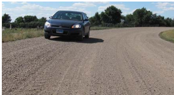
Figure 18. Photo. Super-elevation on sharp curve.
