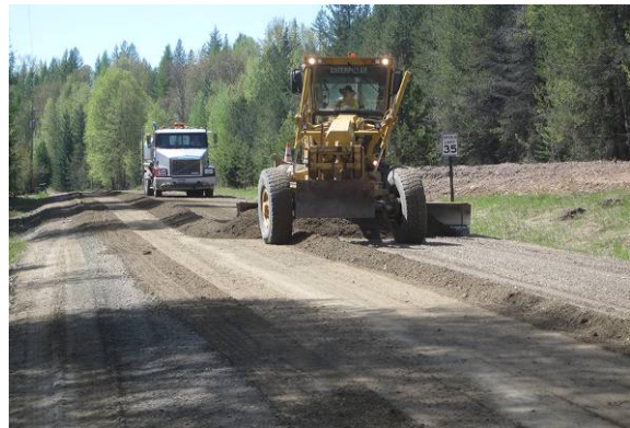
Figure 16. Photo. Maintenance of treated road.
