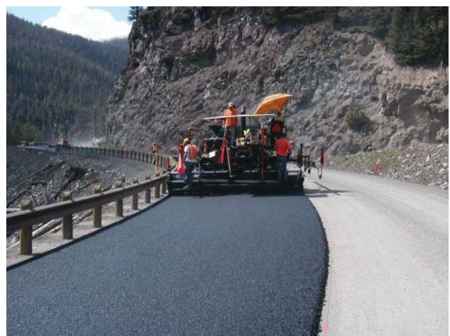
Figure 8 ~ Advera laydown operation.
