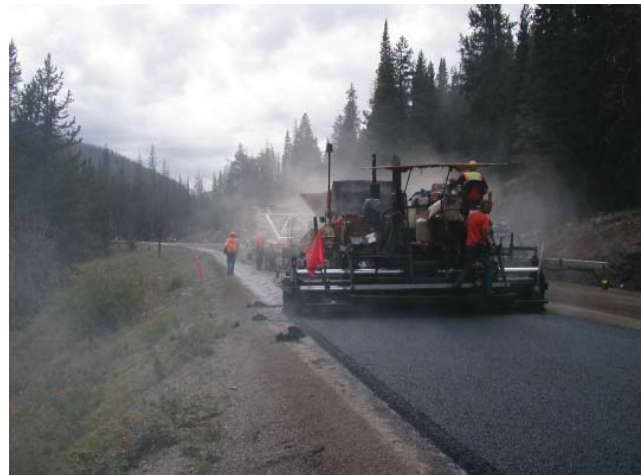
Figure 5 ~ Control mix laydown.
