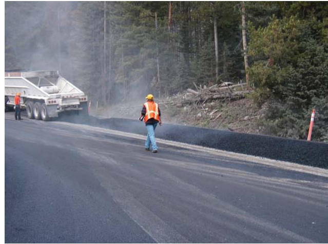
Figure 3 ~ Depositing control mix in windrow.
