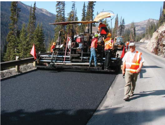
Figure 10 ~ Sasobit laydown operation.
