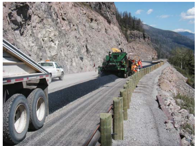
Figure 7 ~ Advera WMA deposited in windrow.
