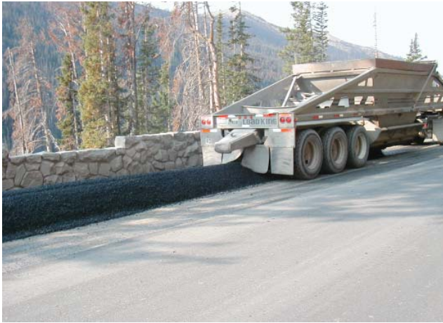
Figure 9 ~ Sasobit deposited in windrow.
