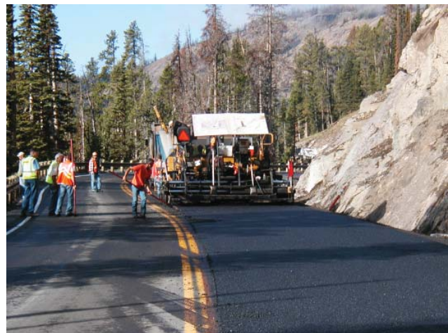
Figure 11 ~ Sasobit laydown operation.
