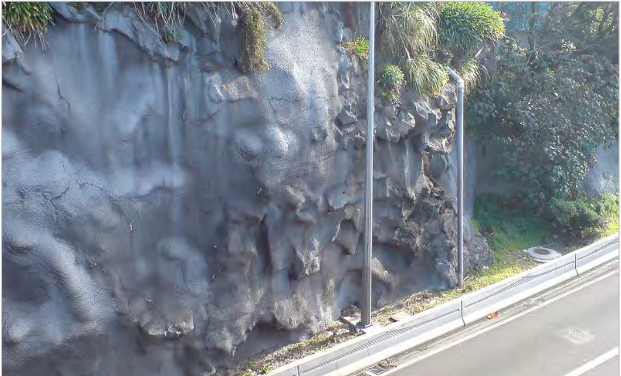
Figure 3-13: Rock fall mitigation using shotcrete to prevent erosion
