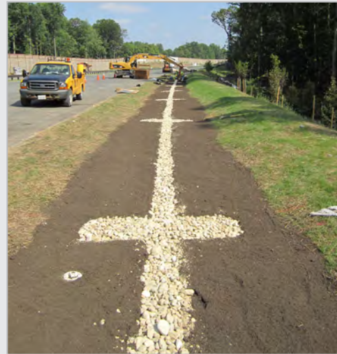
Infiltration swale during construction
