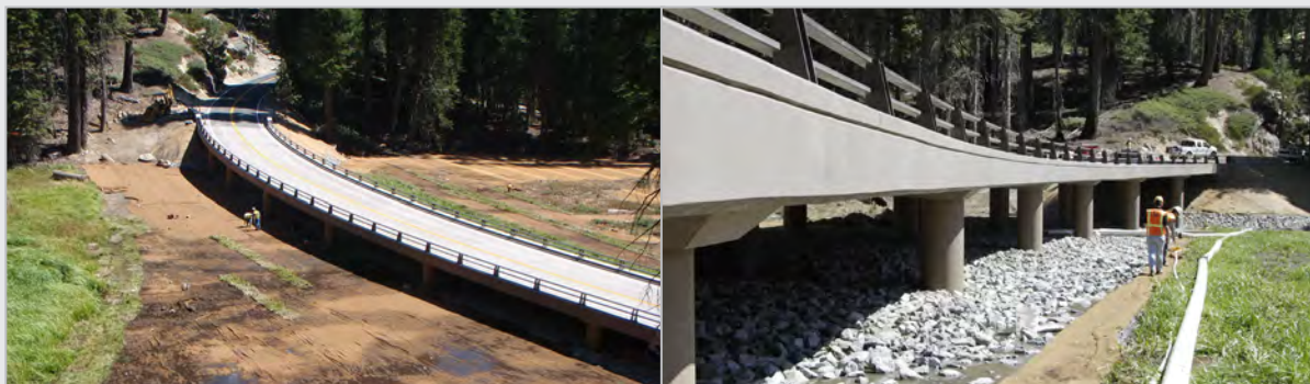
The bridge under construction
