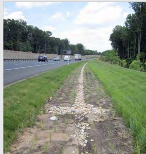
Infiltration swale after construction
