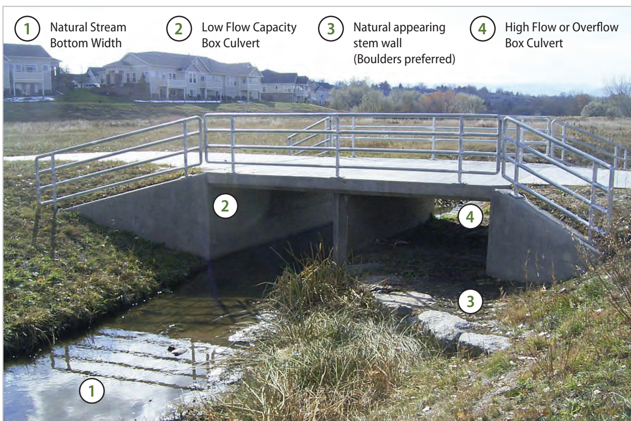
Figure 3-21: Multi-cell box culvert
