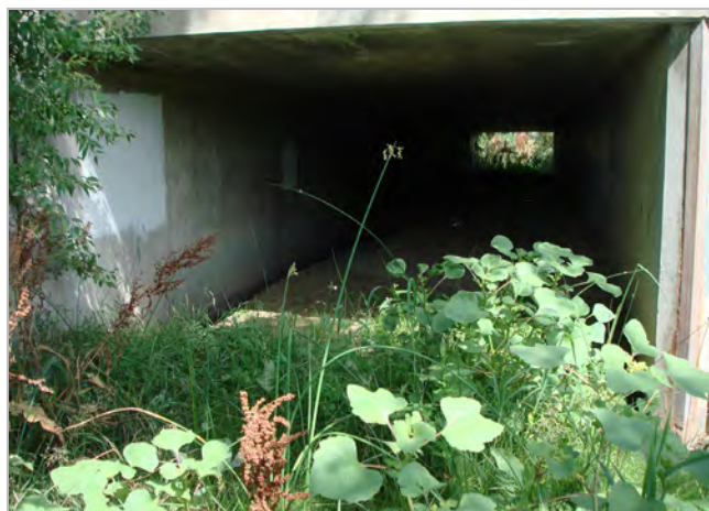
Figure 3-15: Large culvert following major storm event
