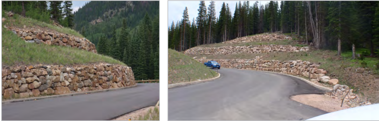
Figure 3-8: Retaining walls enhancing both safety and roadside character
