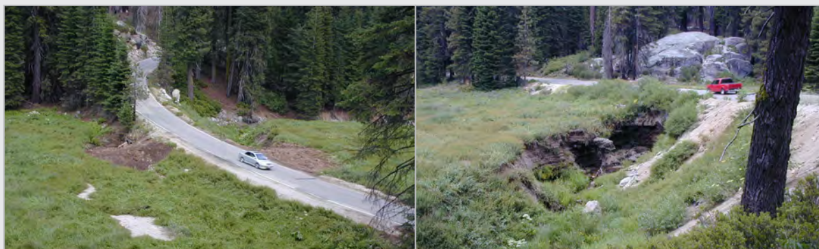
The roadway before project construction
