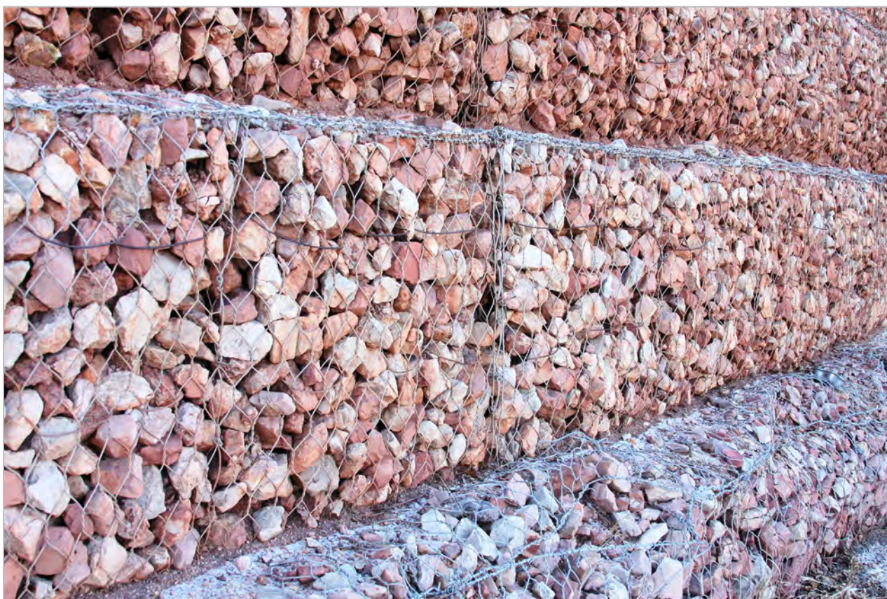
Figure 3-14: Rock wall material (Manitou Springs, Colorado)
