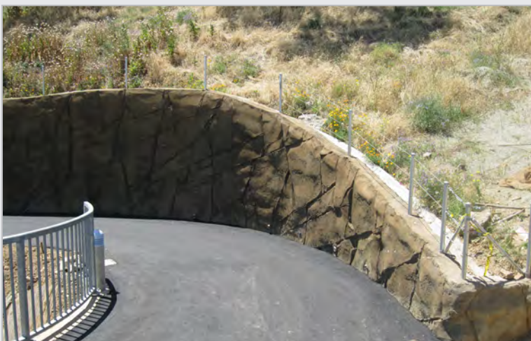
Soil-nail wall system as constructed
