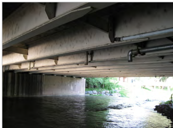
Figure 3-17: Drainage directly into a creek without treatment/infiltration strategies
