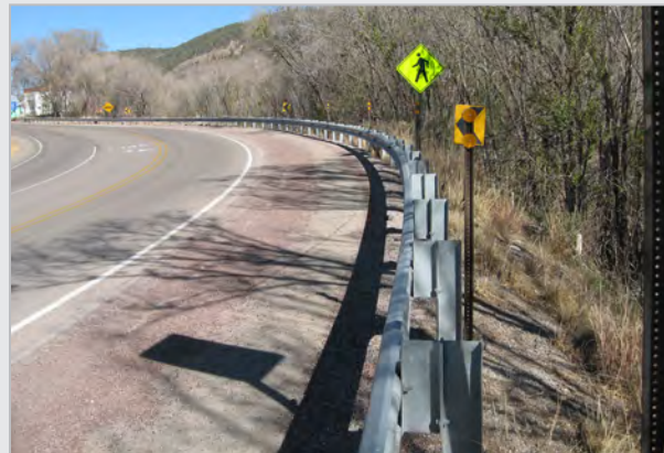
Guardrail placed at steep slope
