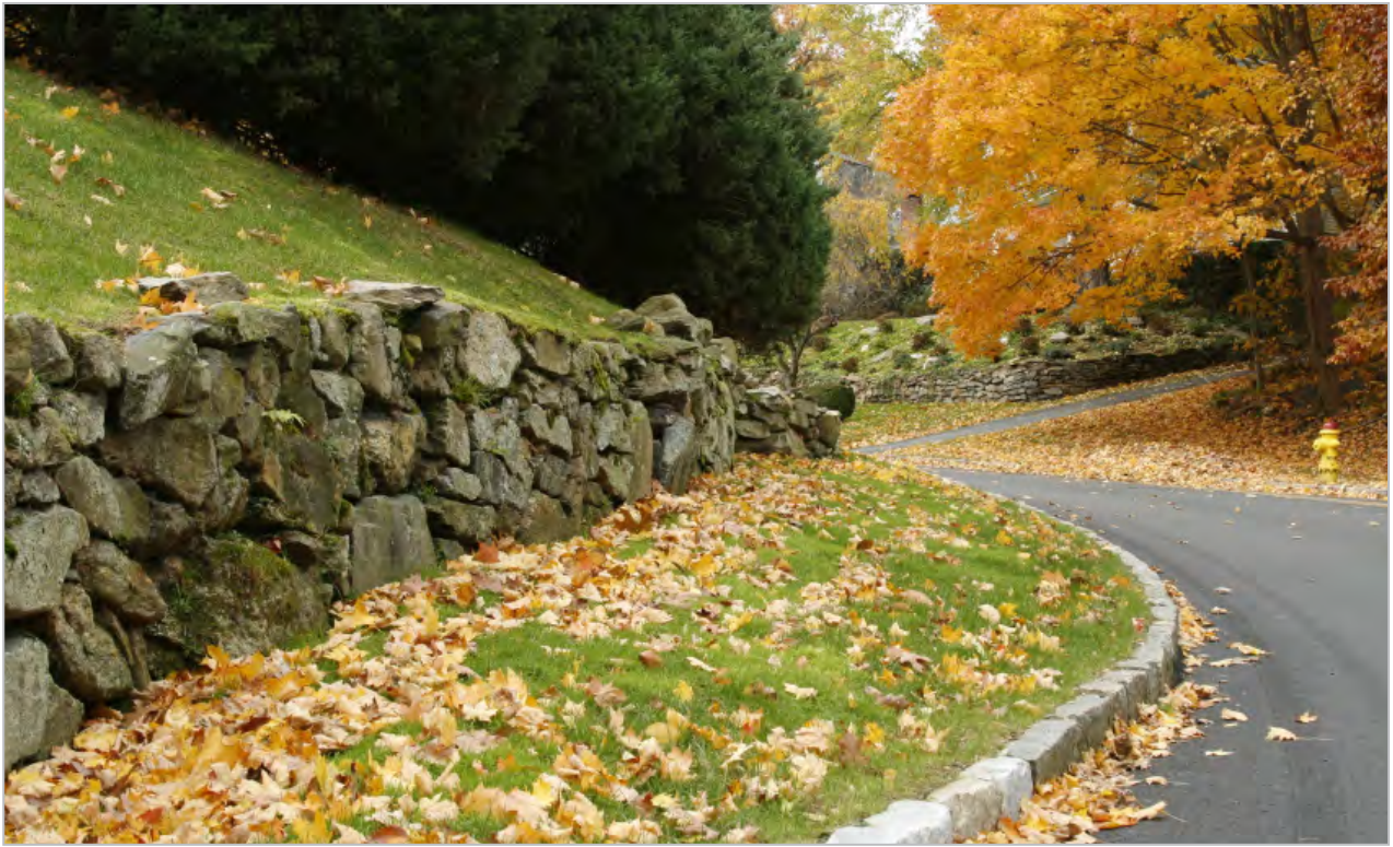
Figure 3-12: Retaining wall enhancing surrounding environment
