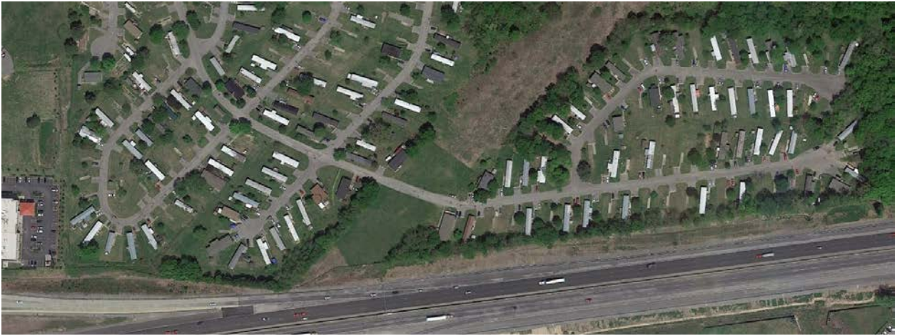
Figure 48. Community for which a noise barrier was proposed by TDOT, Project TDOT-1 (image from www.google.com/maps ).
