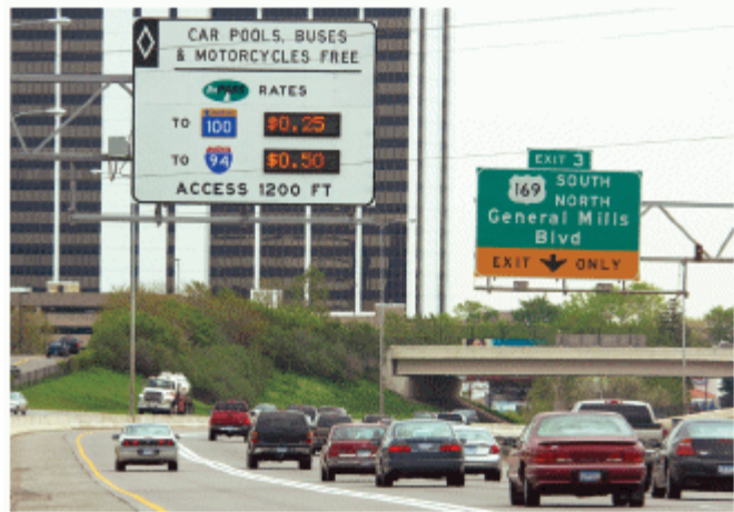
Figure 26. MnPASS Express Lanes (HOT lanes) on I-394
