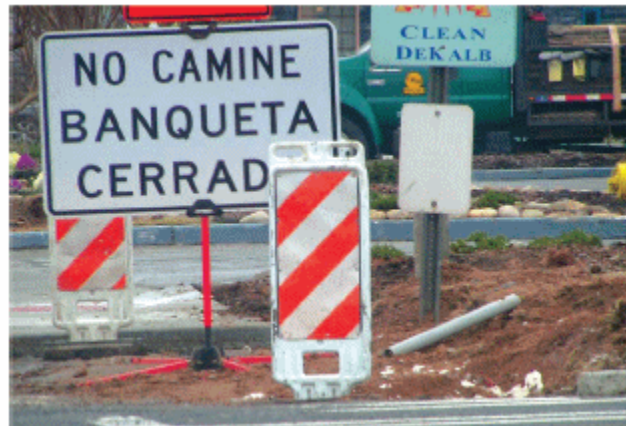
Figure 13. GDOT Construction Signs in Spanish
