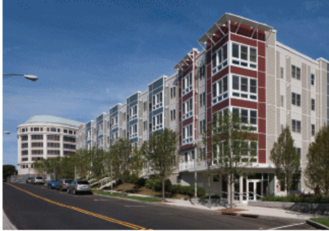
Figure 21. Picture of New Green Affordable Housing Near SITC
