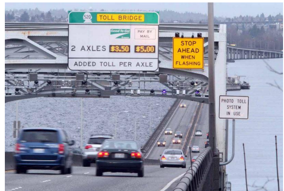
Figure 1: SR 520 Bridge in Seattle, WA, is a fully tolled facility Image Source: Washington State Dept. of Transportation
