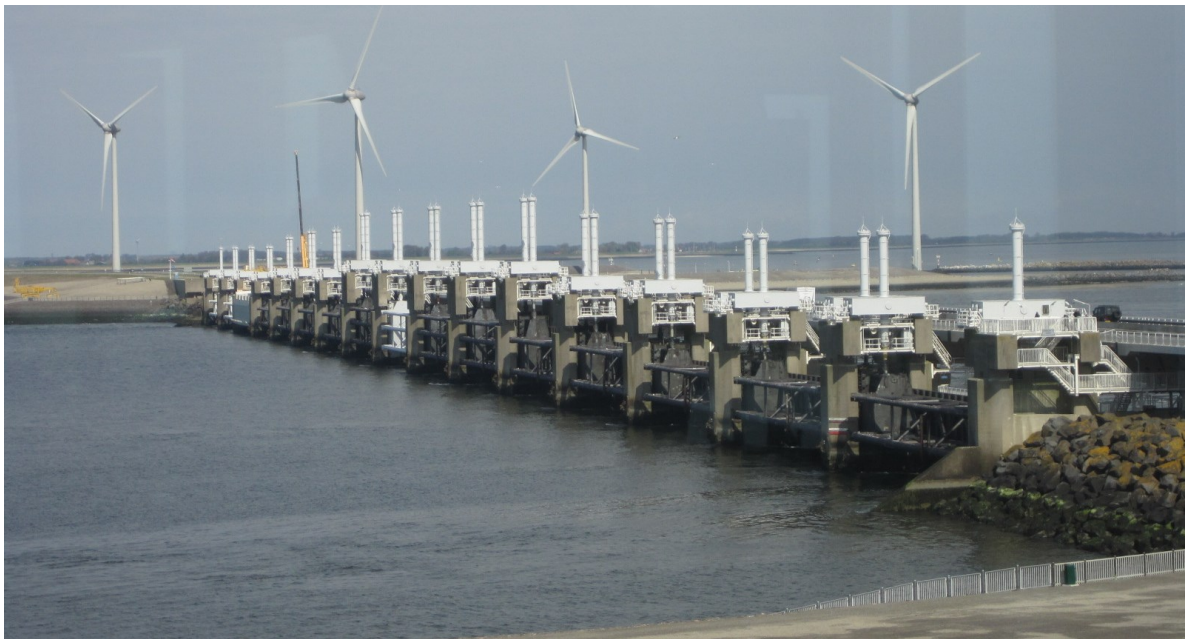
The Eastern Scheldt storm surge barrier in southern Holland. Photo Credit: FHWA
