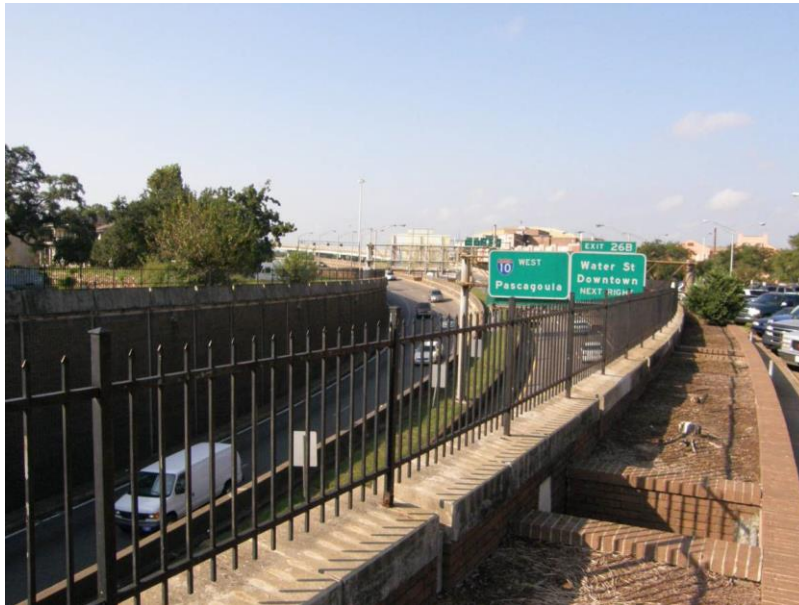
Figure 85: West Portal of the I-10 Tunnel 361
