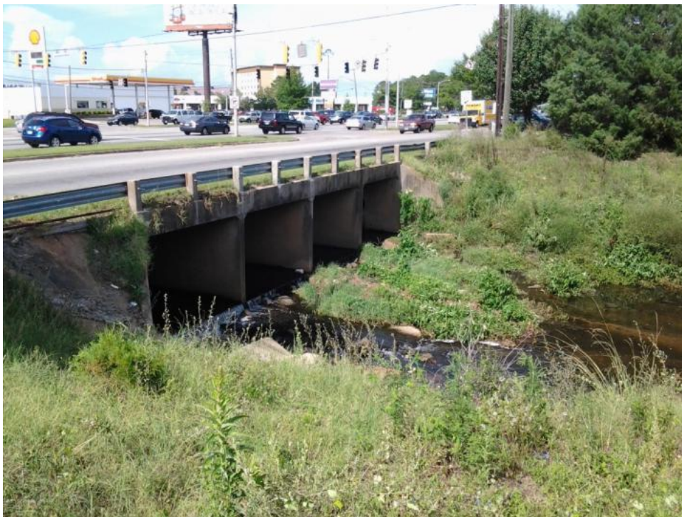
Figure 13: Photo of the Airport Boulevard Culvert over Montlimar Creek, Downstream Side
