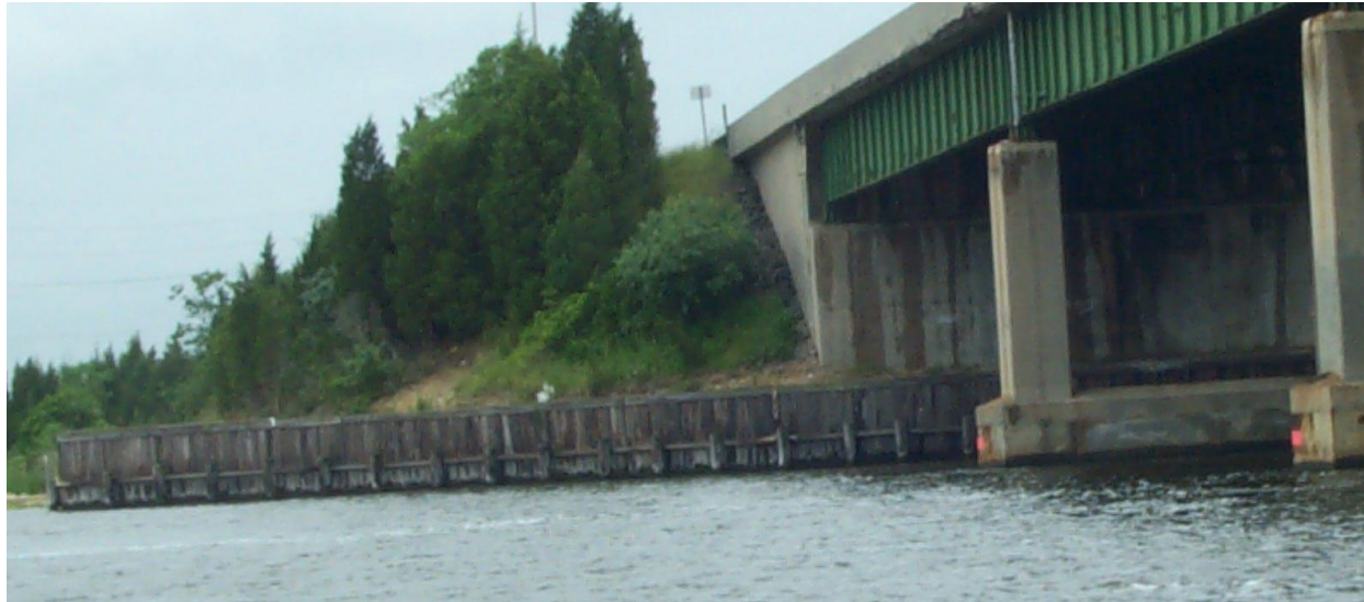
Figure 54: Example of Typical Timber Bulkhead Protection at a Highway Bridge Abutment 180
