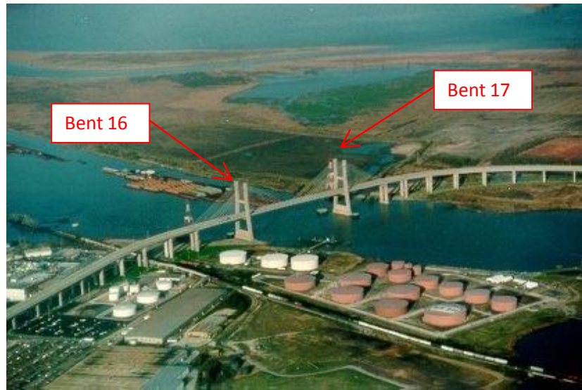
Figure 32: Image of the Cochrane-Africatown USA Bridge Showing the Section of Analysis between Bents 16 and 17 97
