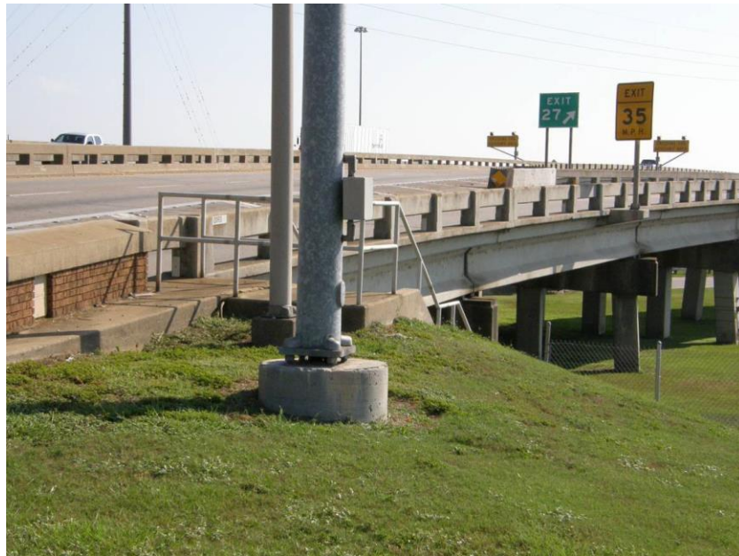
Figure 86: Portion of I-10 Immediately East of the I-10 Tunnel Portal 375
