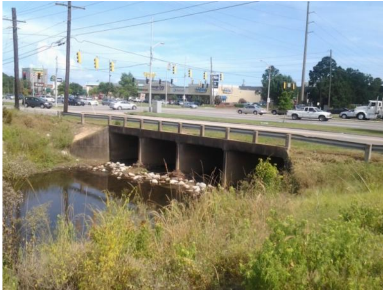
Figure 6: Photo of the Airport Boulevard Culvert over Montlimar Creek, Upstream Side
