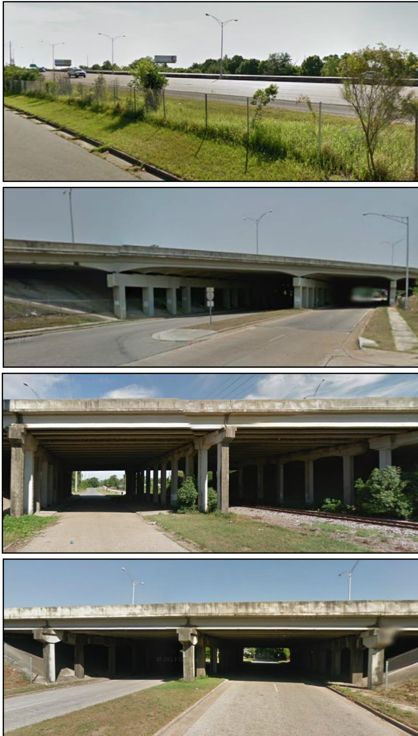
Figure 75: Study Area Images (Top to Bottom: I-10 Roadway Looking East from North of the Embankment Near the Low Point, Broad St. Underpass, Tennessee St. and Railroad Underpass, and Warren St. Underpass Looking North) 314
