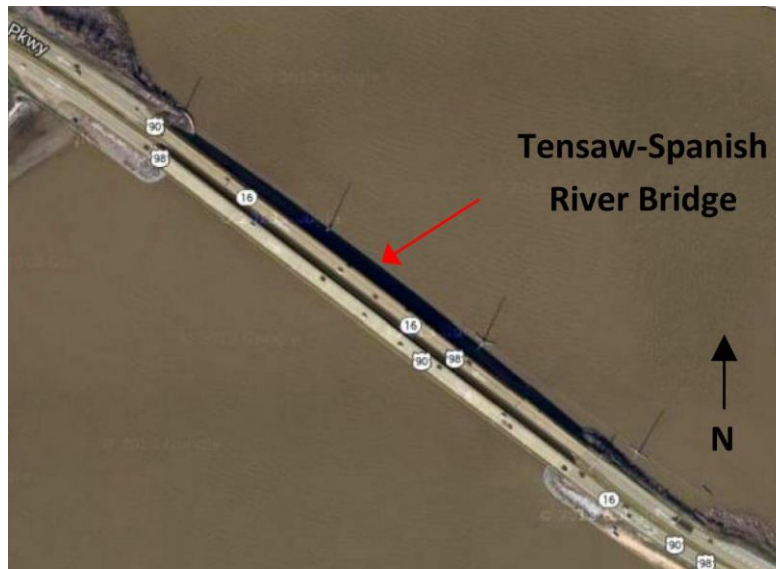
Figure 47: Aerial Image of the US 90/98 Tensaw-Spanish River Bridge 170
