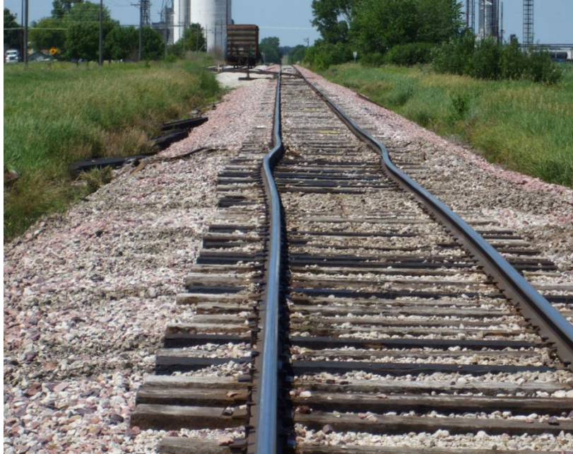
Figure 97: Example of a Hot Weather Sun Kink 459
