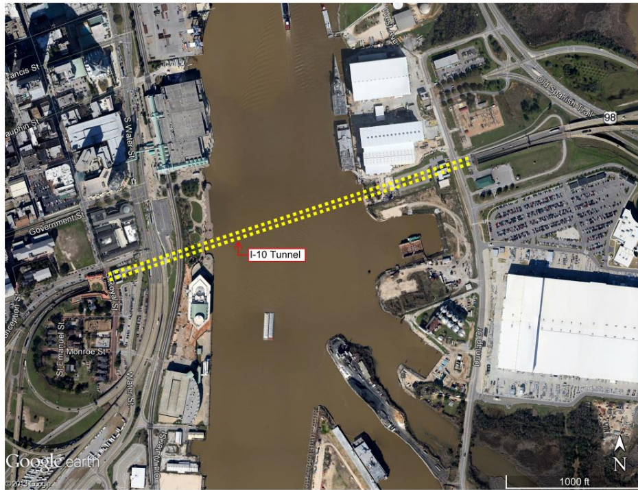
Figure 84: Aerial Photograph of the I-10 Tunnel 360
