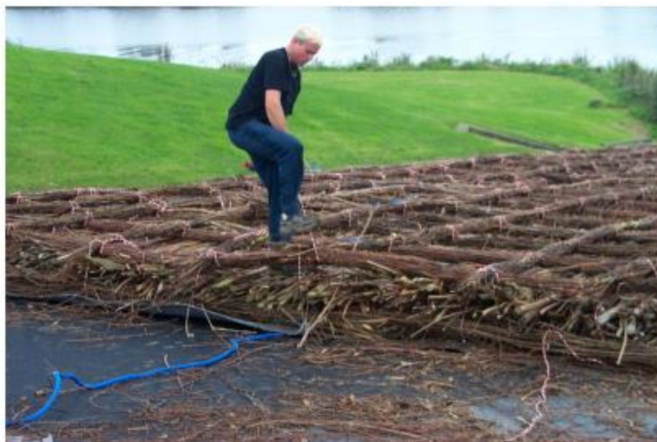
Figure 53: Representative Willow Mattress Pad (Assembly Prior to Submergence) 179
