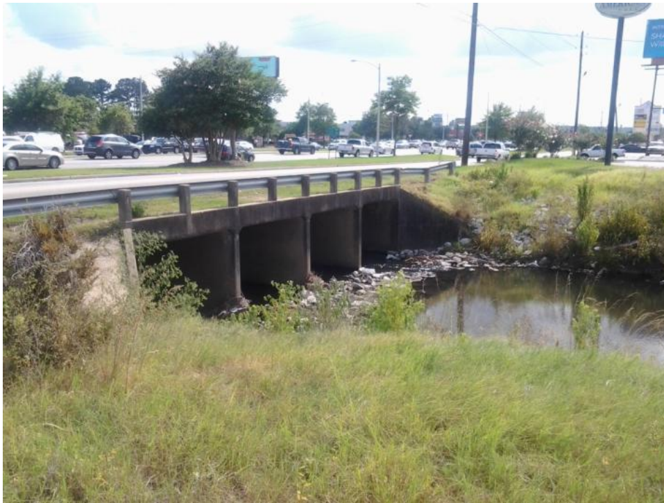
Figure 12: Photo of the Airport Boulevard Culvert over Montlimar Creek, Upstream Side
