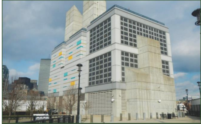
FIGURE 32: CENTRAL ARTERY TUNNEL VENTILATION BUILDING.
