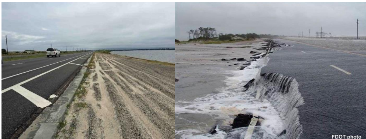
FIGURE 13: COASTAL CLIMATE CHANGE ADAPTATION MEASURES WILL BE SIMILAR TO COASTAL ENGINEERING STRATEGIES FOR IMPROVING RESILIENCE TO TODAY'S EXTREME WEATHER EVENTS.
