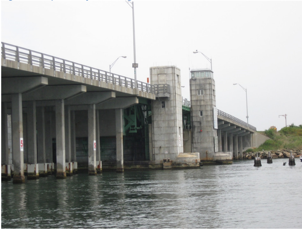
Figure 4: Loop Parkway Over Long Creek – South Side
