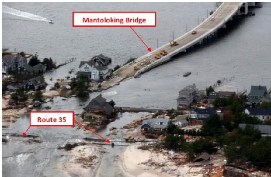
Figure 12: Damage from Hurricane Sandy to Mantoloking Bridge and Route 35
