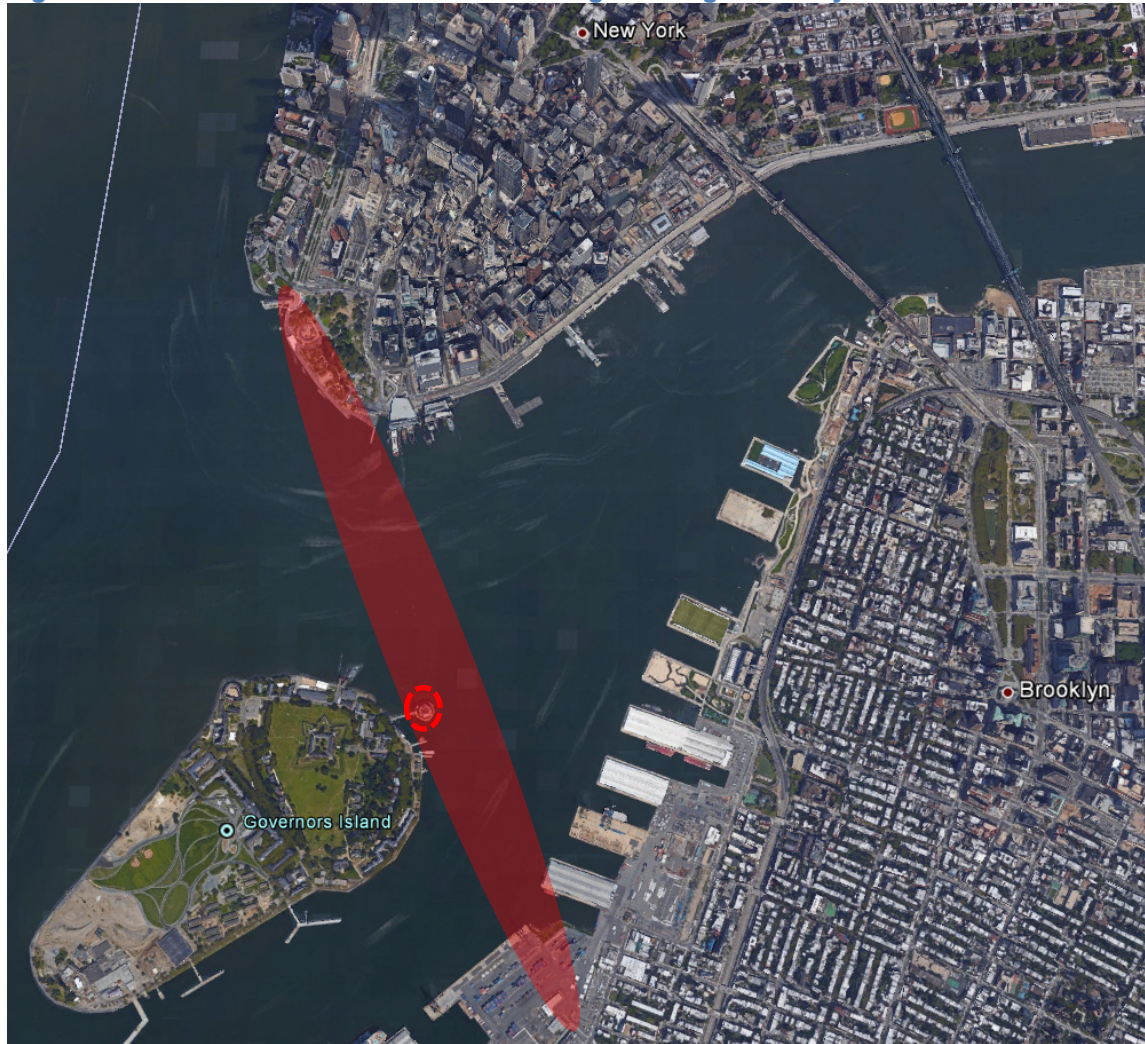
Figure 2: Governors Island Ventilation Building and Hugh L. Carey Tunnel
