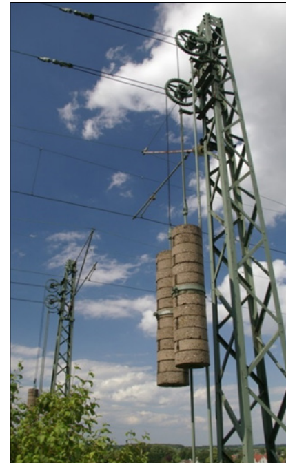
Figure 9: Constant Tension Catenary System
