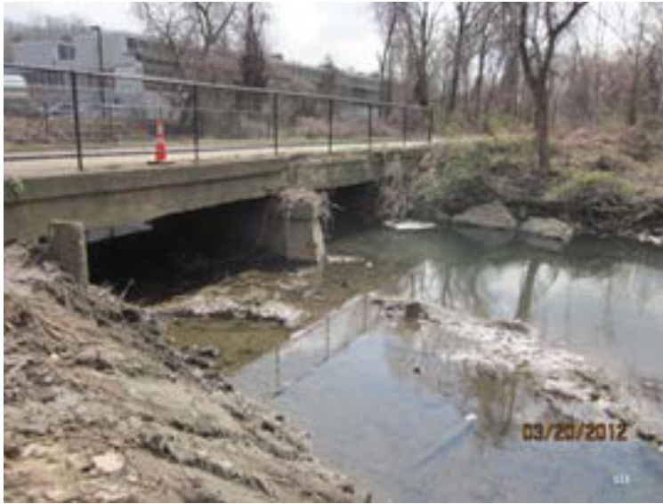
Figure 4: Culverts after debris removal
