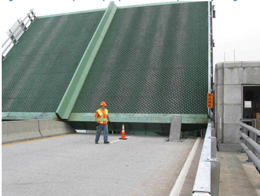
Figure 3: Bascule span in open position on Loop Parkway Bridge
