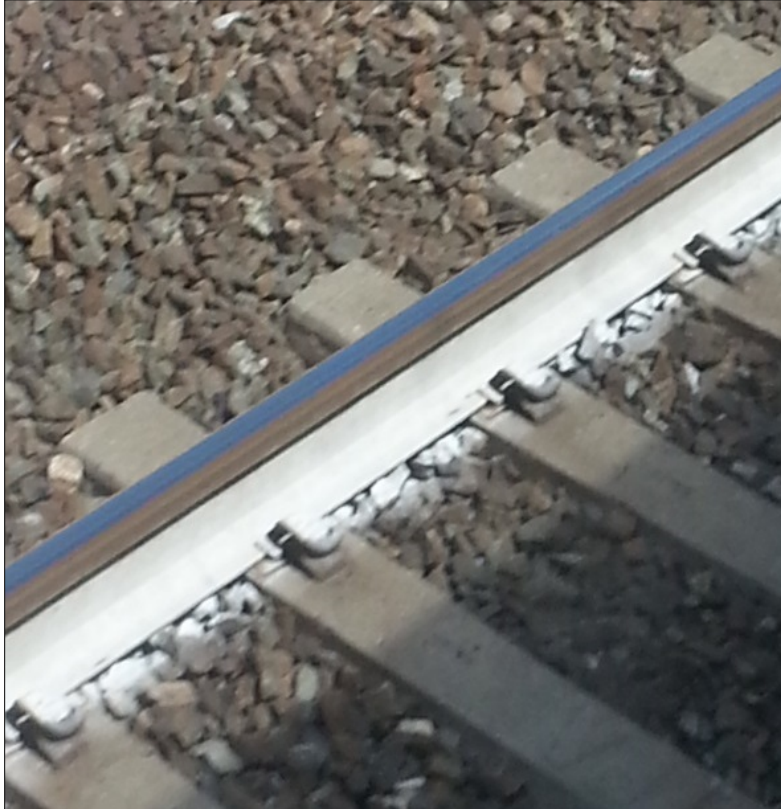
Figure 8: Running Rail with Web Painted White in Northern Italy
