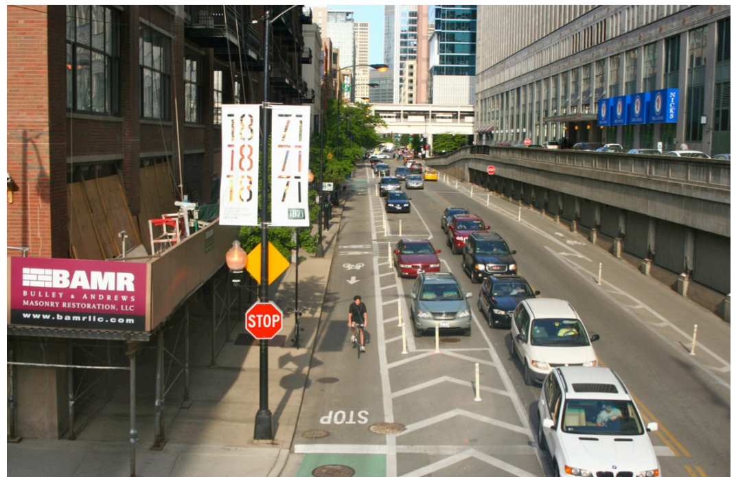
On Kinzie Street in Chicago, parked cars and flexible delineator posts on both sides of the street separate the bike lanes from traffic. (Source: City of Chicago)
