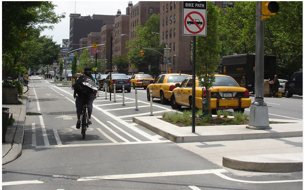
Raised curb islands at intersections combined with flexible delineator posts and parked cars midblock on 9th Avenue in New York City, NY (Source: NYC DOT)
