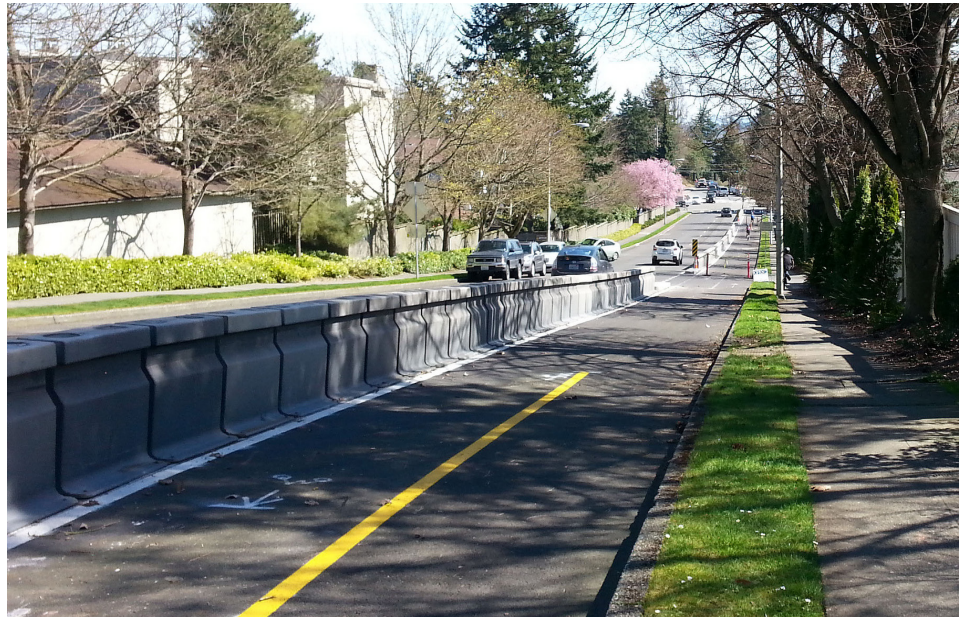
Seattle, WA. (Source: Seattle DOT)
