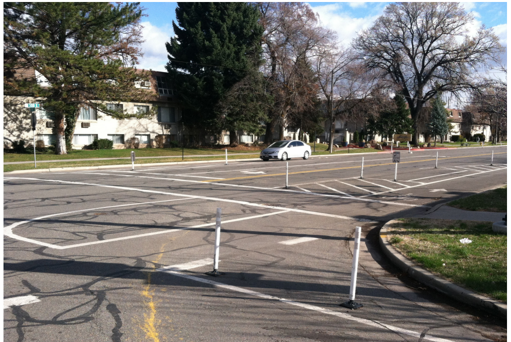
Salt Lake City's 300 East separated bike lane was installed using PBPD with inexpensive materials (Source: City of Salt Lake City)
