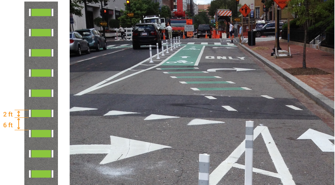
Green paint across a mixing zone opening on M Street NW in Washington, DC (Source: Jason Broehm)
