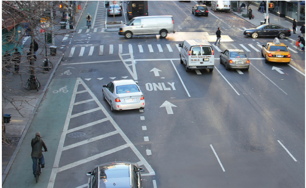
A separated bike lane, shorter crossing distances, and a dedicated bus lane along 1st Avenue, New York City (Source: NYCDOT)
