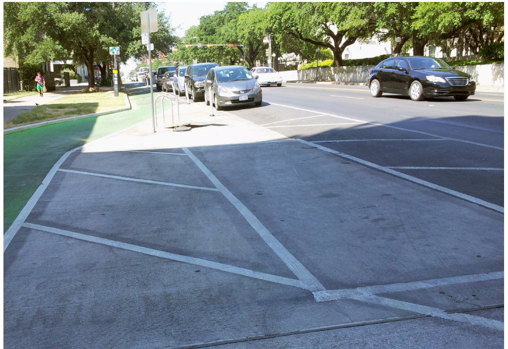
A dedicated accessible parking space with access aisle in Austin, TX. (Source: Kelly Blume)
