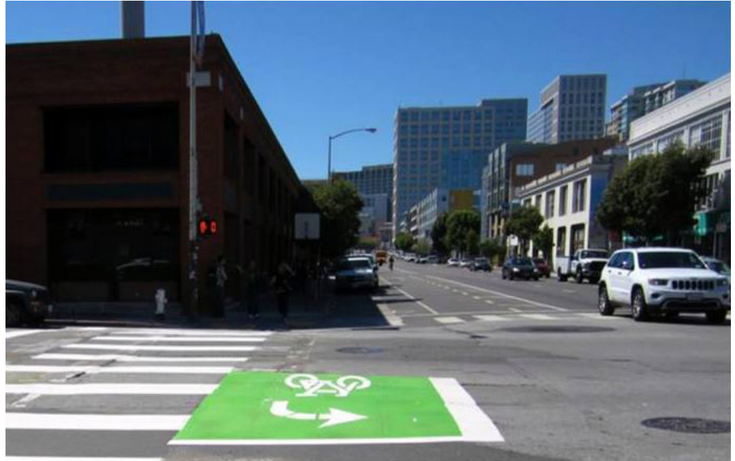
An example of a left-turn queue box used on a bike lane in San Francisco. (Source: San Francisco Municipal Transportation Agency)
