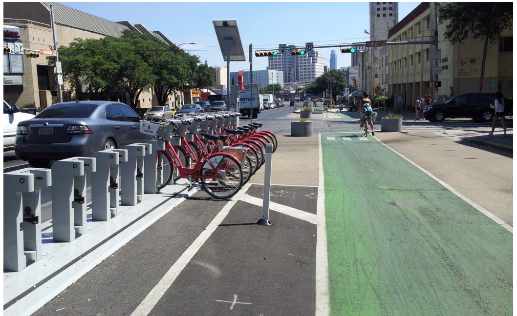
A B-Cycle docking station provides physical separation within the buffer space in Austin, TX, between the separated bike lane and vehicle travel lanes. (Source: City of Austin)
