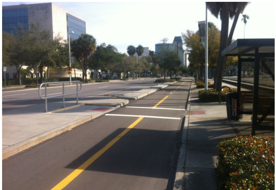
Platform island bus stop and 1st Avenue South separated bike lane in St. Petersburg, FL. (Source: Rory Rowan)
