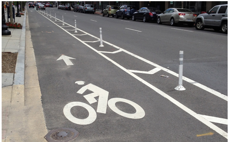
Inexpensive treatment with flexible delineator posts on L Street, Washington DC (Source: DDOT)
