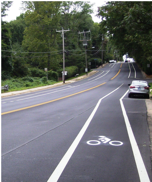
Bike lanes were added Sherwood Hill Lane in Alexandria, VA, by narrowing unnecessarily wide parking lanes.
