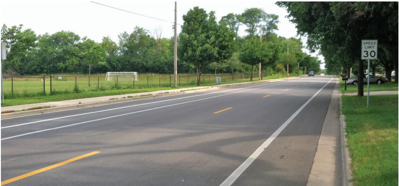
Bike Lanes were added to Portage Road in Madison, WI, by clearly defining overly wide shared travel/parking lanes.
