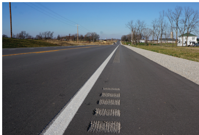
Highway 26 near Rosendale, WI, was recently resurfaced with 5-foot wide shoulders and narrow rumble strips that leave four feet of clear pavement to the right of the rumble strip.
