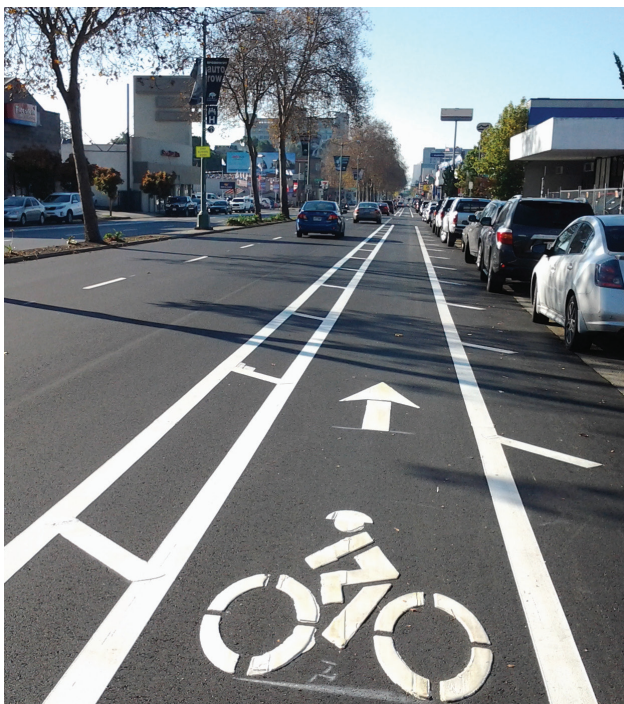
Buffered bike lanes were added to Broadway in Oakland, CA, during a resurfacing project by removing one travel lane in each direction.
