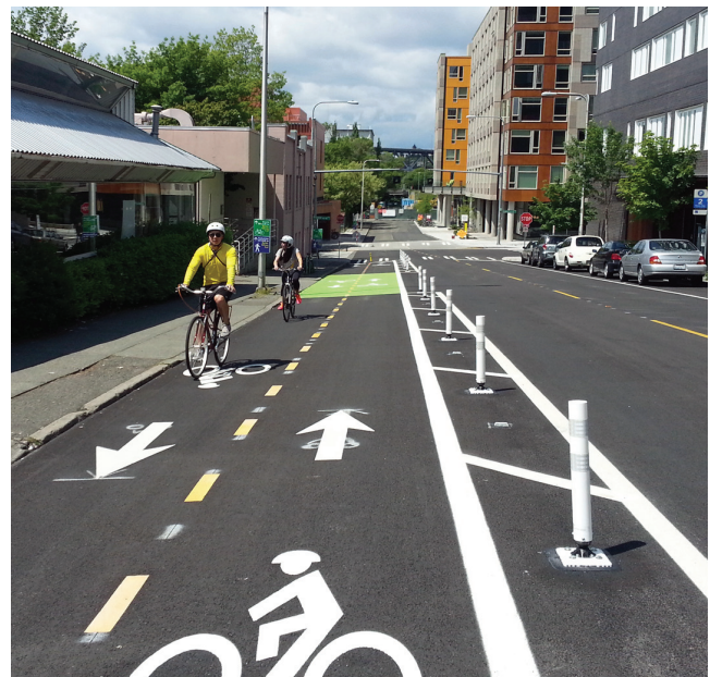
This two-way separated bike lane was added during a resurfacing project on NE 40th Street in Seattle, WA.
