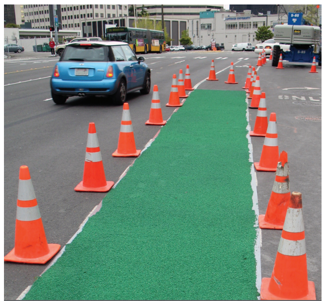
A marking plan is essential to ensure bikeways are marked as intended following a resurfacing. Green pavement markings have received interim approval from FHWA, but agencies must seek approval from FHWA prior to using green markings.
