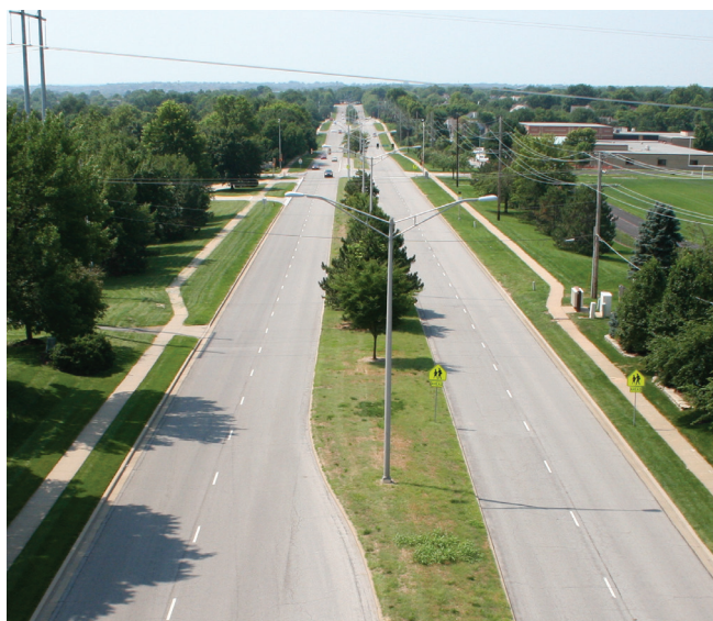
Bicycle lanes were added to Switzer Road in Overland Park, KS, during a resurfacing project by narrowing the travel lanes.
