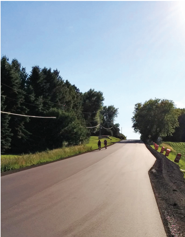
A paved shoulder has been added to Whalen Road in Fitchburg, WI, in uphill directions as part of a resurfacing project; markings have not yet been added.
