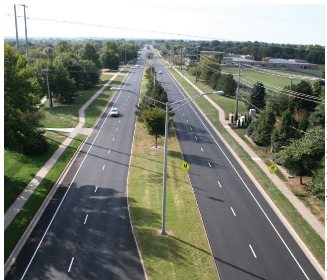
Bicycle lanes were added to Switzer Road in Overland Park, KS, during a resurfacing project by narrowing the travel lanes.
