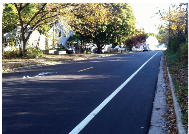
Bluff Street in Madison, WI, had a bicycle lane installed in the uphill direction and shared lane markings in the downhill direction during a resurfacing project. This configuration allowed parking to be preserved on one side of the street.
