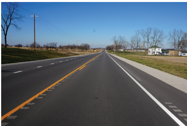
Highway 26 near Rosendale, WI, was recently resurfaced with 5-foot wide shoulders and narrow rumble strips that leave four feet of clear pavement to the right of the rumble strip.
