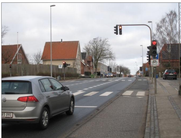
Figure 8. Bicycle Exemption from Traffic Signal Control at T-Intersection, Odense, Denmark
