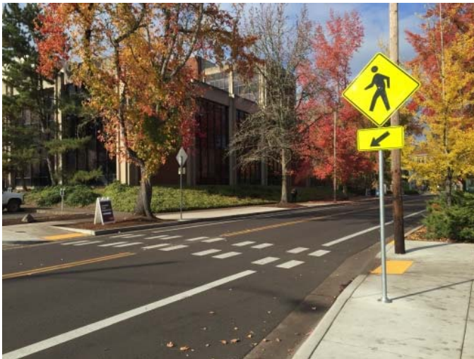
Exhibit 48. SW 15 TH STREET LOOKING NORTH (TOP), GRAPHIC SHOWING AERIAL VIEW (BOTTOM)
