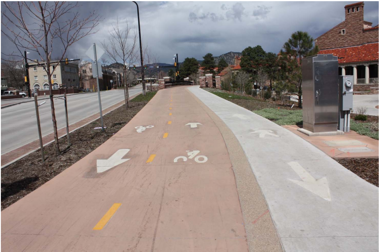
Exhibit 21. BROADWAY SIDEPATH LOOKING EAST
