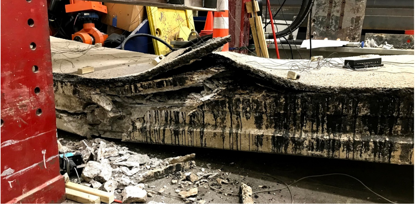
Figure 11. Photo. A picture of the flexural failure at midspan.
