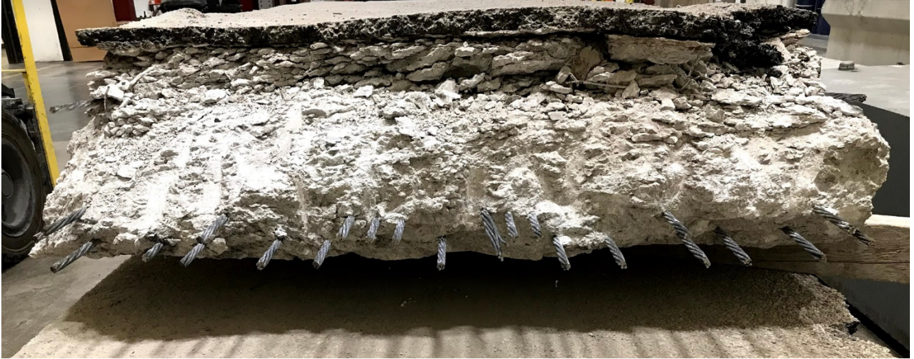
Figure 15. Photo. Cross-section of the beam specimen after cutting prestressing strands. Note that the configuration of the strands is different than shown in Figure 4.
