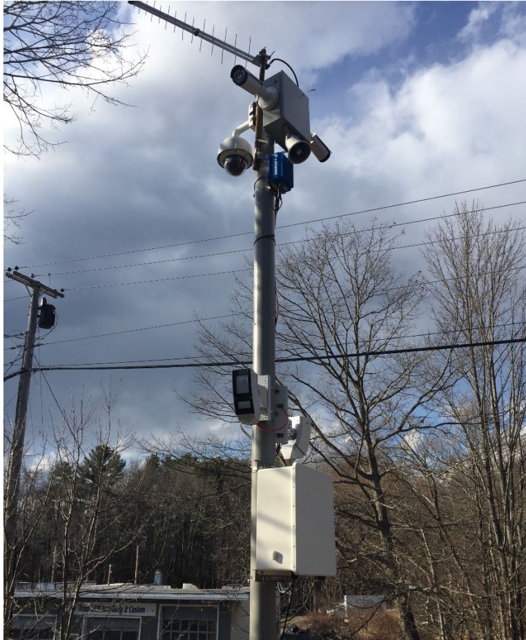
Figure 10 – Jordan Avenue Pole with Optex Sensors
