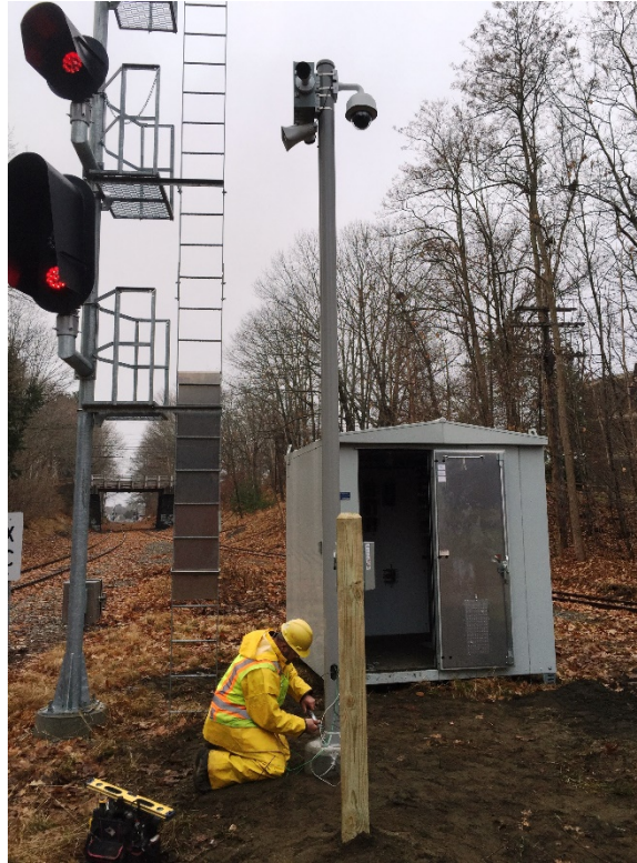
Figure 4 – Rock Junction Camera Pole
