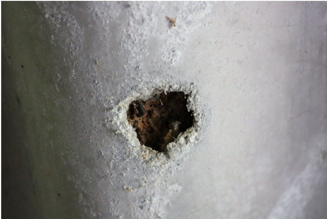
Photo 18 Close-up view of through-wall pit.
