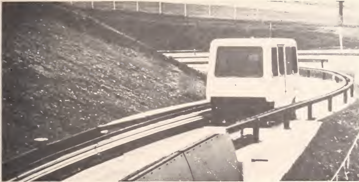
A View Along the Morgantown Guideway.
