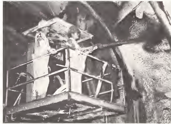
The Use of Shotcrete is an Example of a Cost Saving Construction Technique Being Investigated.
