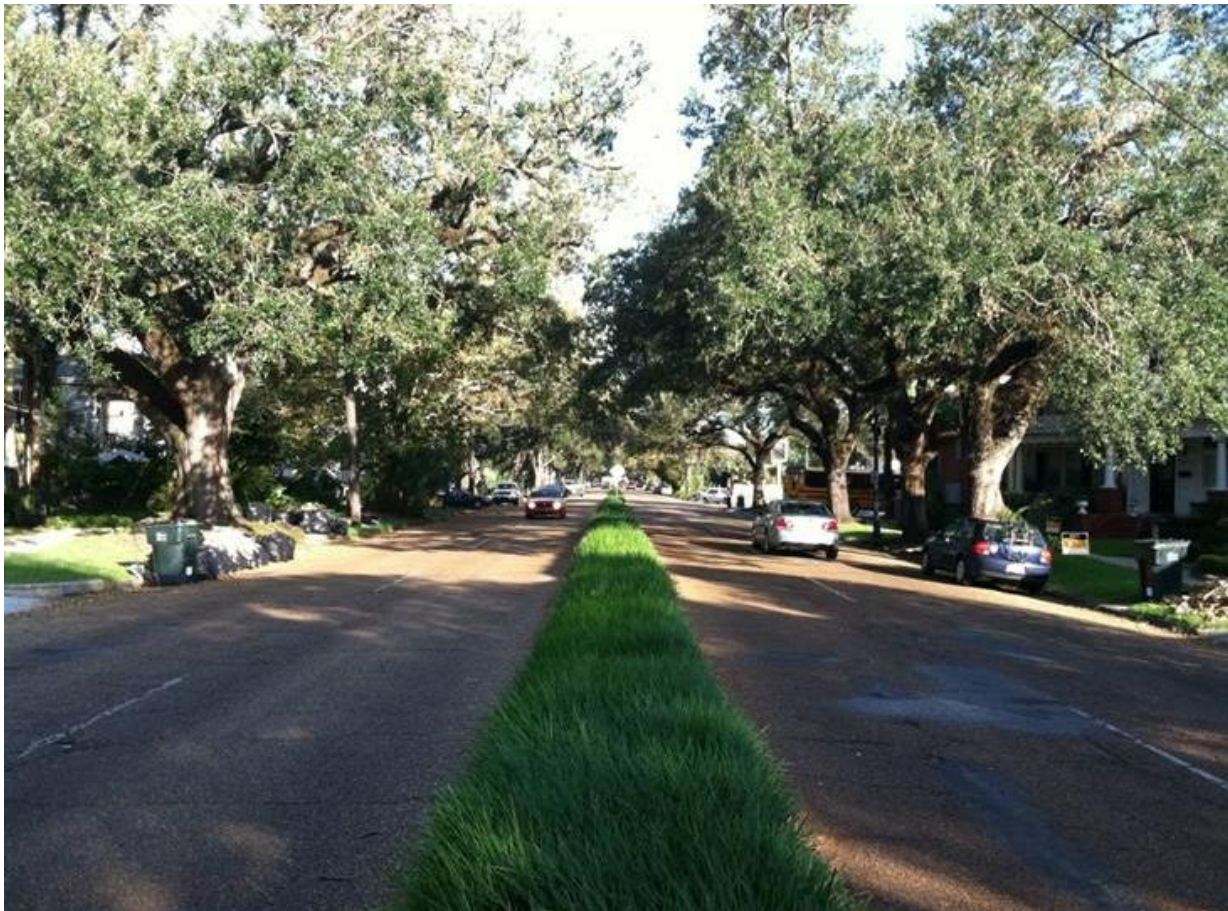
Figure 18. Prior to the project, Esplanade Avenue's narrow lanes and frequent driveways, combined with high speeds, made the corridor uncomfortable for pedestrians and bicyclists. Image courtesy of FHWA Louisiana Division Office.
