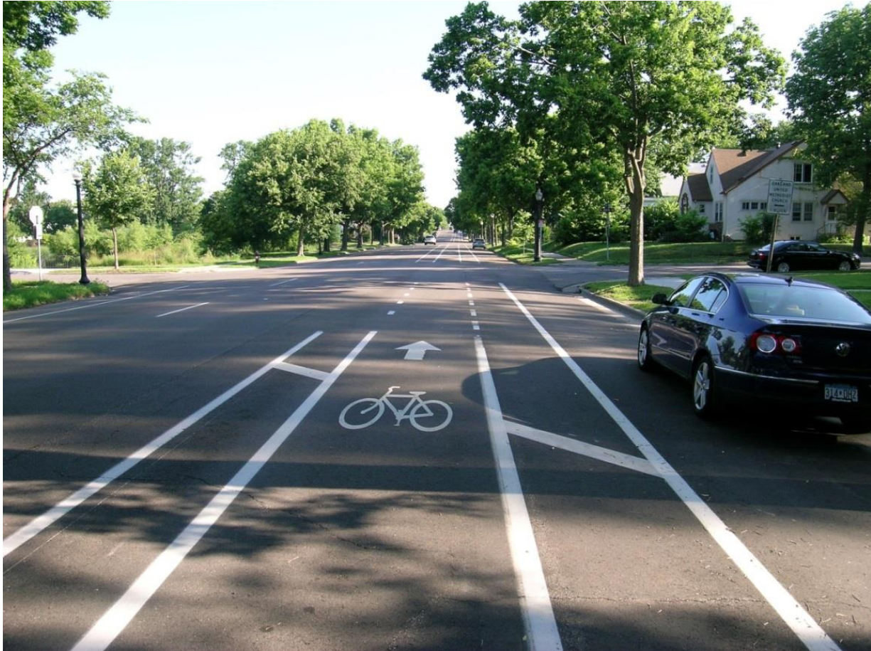
Figure 27. Buffered bike lanes, like the ones installed in Minneapolis, Minnesota, are excellent examples of low cost network improvements for bicyclists. Image courtesy of the FHWA Minnesota Division Office
