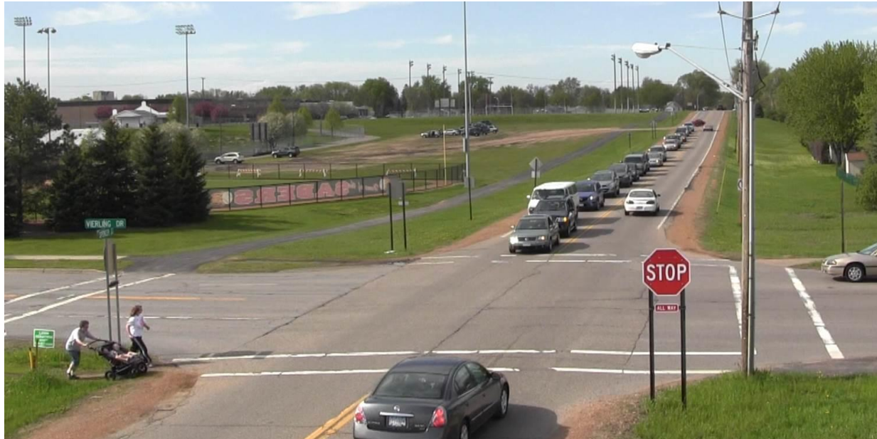
Figure 31. Prior to the installation of the roundabout, the stop-controlled intersection had a history of long delays. Image courtesy of the FHWA Minnesota Division Office
