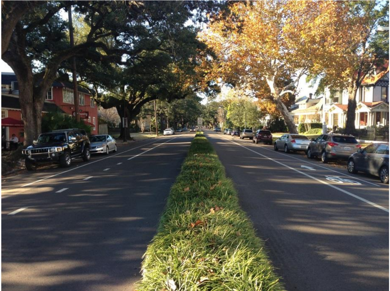
Figure 19. The resulting road diet improved comfort for nonmotorized users, evident in the increases in bicycling and walking along the corridor following the project. Image courtesy of FHWA Louisiana Division Office.
