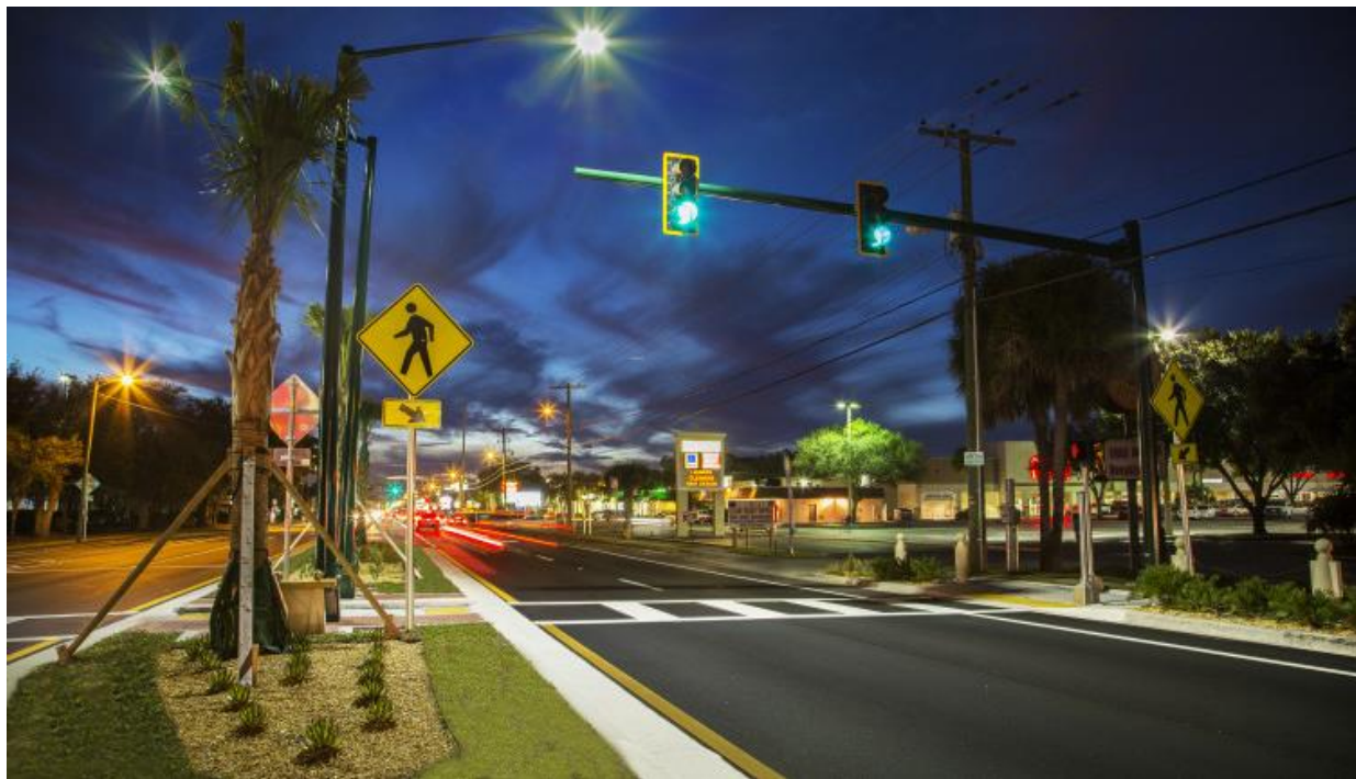
Figure 17. One of the new signalized pedestrian crossings installed on Fletcher Avenue. Image courtesy of David Conner and Associates.
