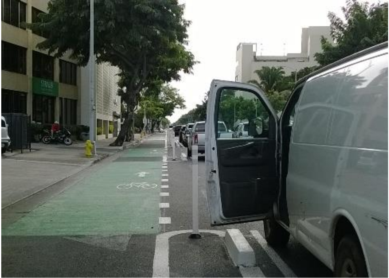
Figure 29. The bicycle lane provides space for a car door to open in the parking area without posing a risk to cyclists. Image courtesy of Hawaii Department of Transportation (HDOT).
