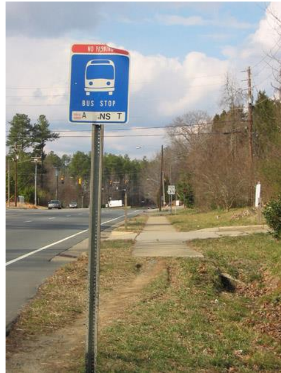
Figure 1. The sidewalk stops short of the bus stop location. Image courtesy of the PBIC Image Library (Photographer: Laura Sandt)
