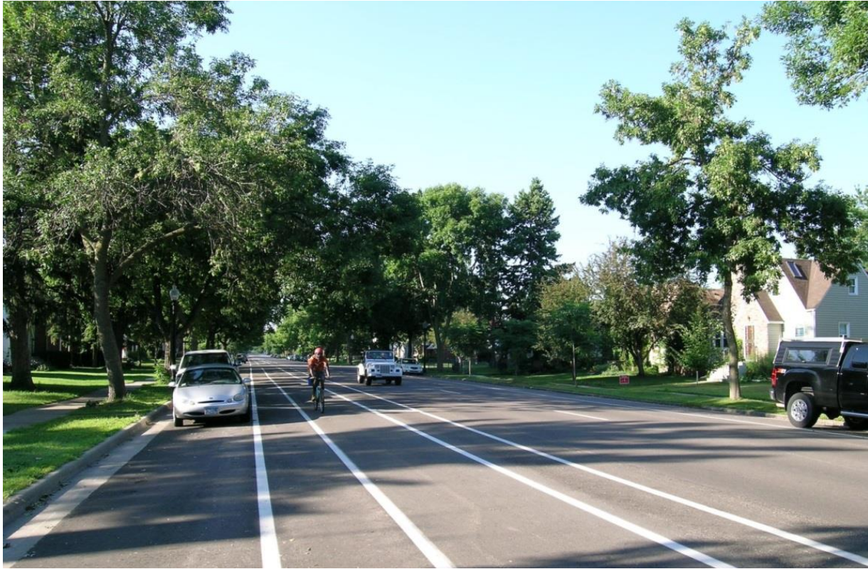
Figure 28. A cyclist riding in the buffered bicycle lane. Image courtesy of the FHWA Minnesota Division Office
