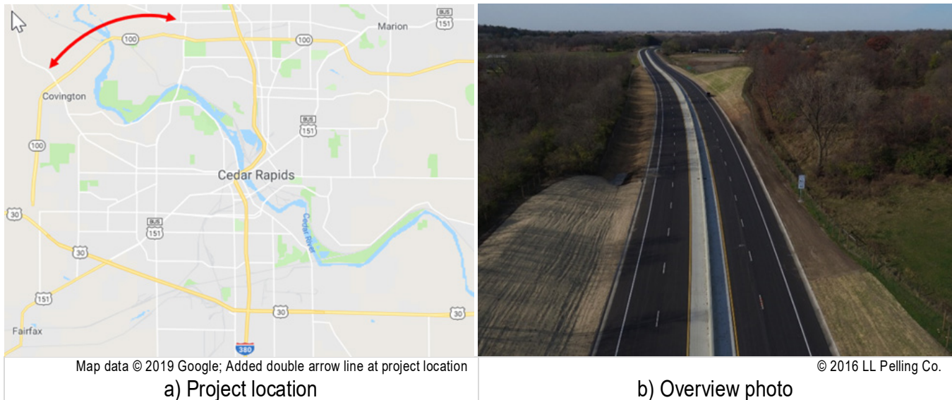
Figure 1. Iowa State Highway 100 project near Cedar Rapids.
